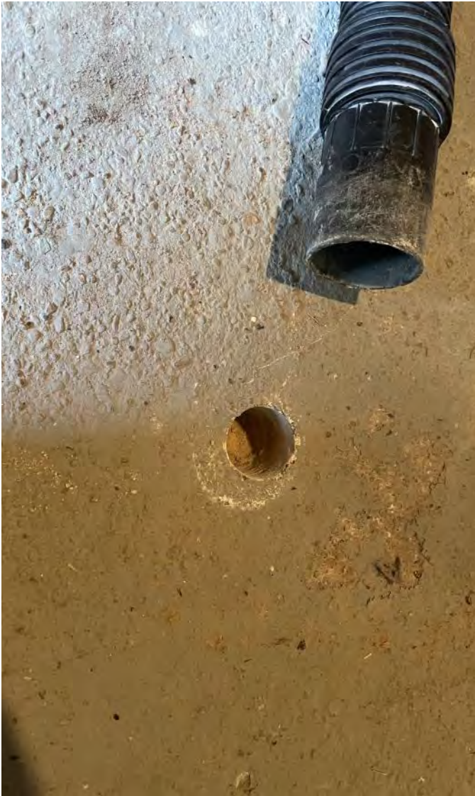
Photo 1: 1 1/2" diameter hole drilled through the concrete floor slab. Photograph taken on June 9, 2023.
