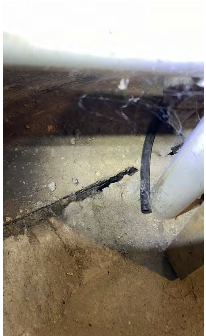
Photo 2: Perimeter joint around the exterior walls of the basement. Photograph taken on May 22, 2023.
