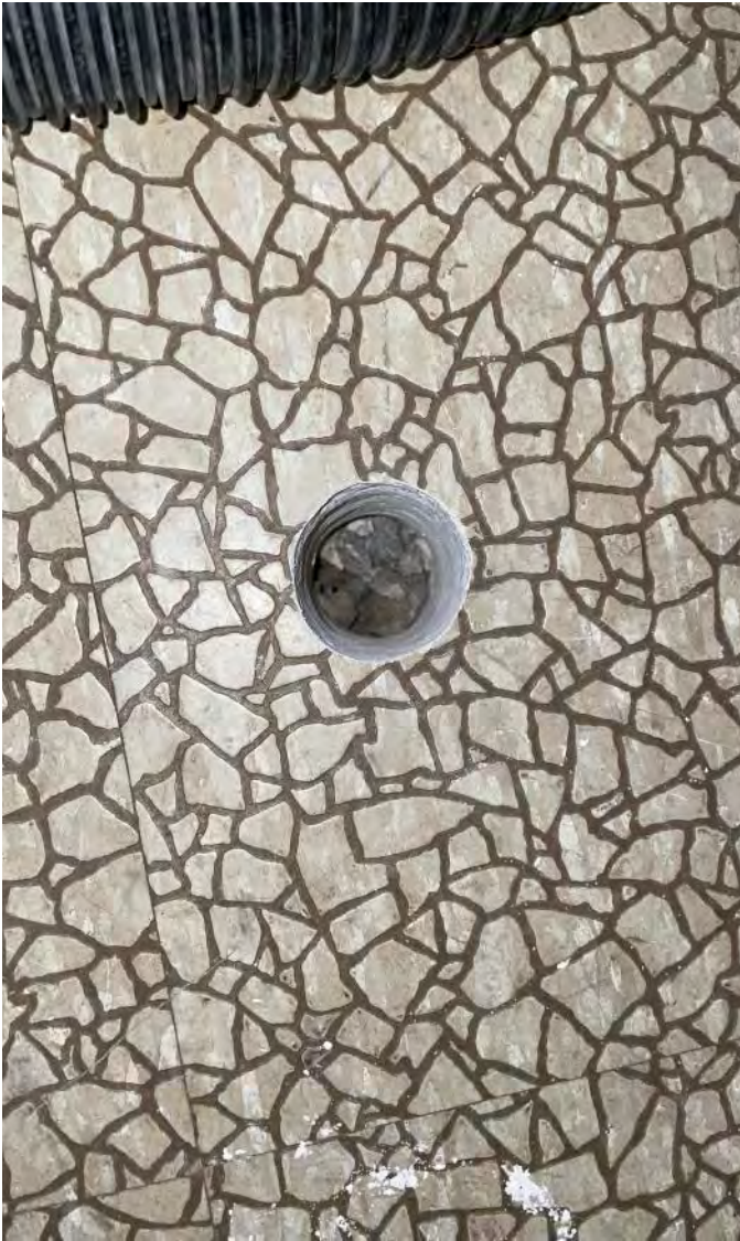
Photo 1: 1 1/2" diameter hole drilled through the concrete floor slab. Photograph taken on June 12, 2023.
