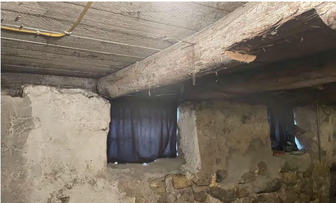
Photo 4: Wooden beams within basement of home. Photograph taken on May 19, 2023.
