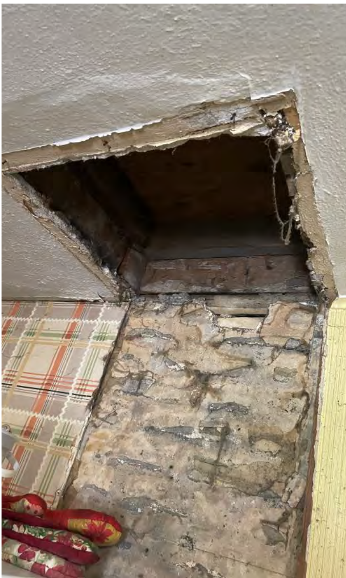
Photo 4: Location of former chimney on the first floor. Photograph taken on May 19, 2023.
