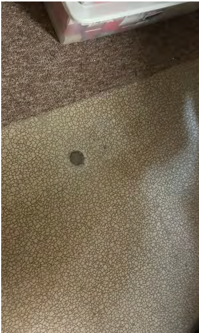
Photo 5: Abandoned sub-slab sample point on April 19, 2024.
