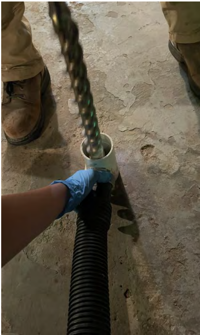
Photo 1: Drilling 1 1/2" diameter hole through the concrete floor slab using a hammer drill and a t-fitting installed on to the shop vacuum. Photograph taken on June 9, 2023.
