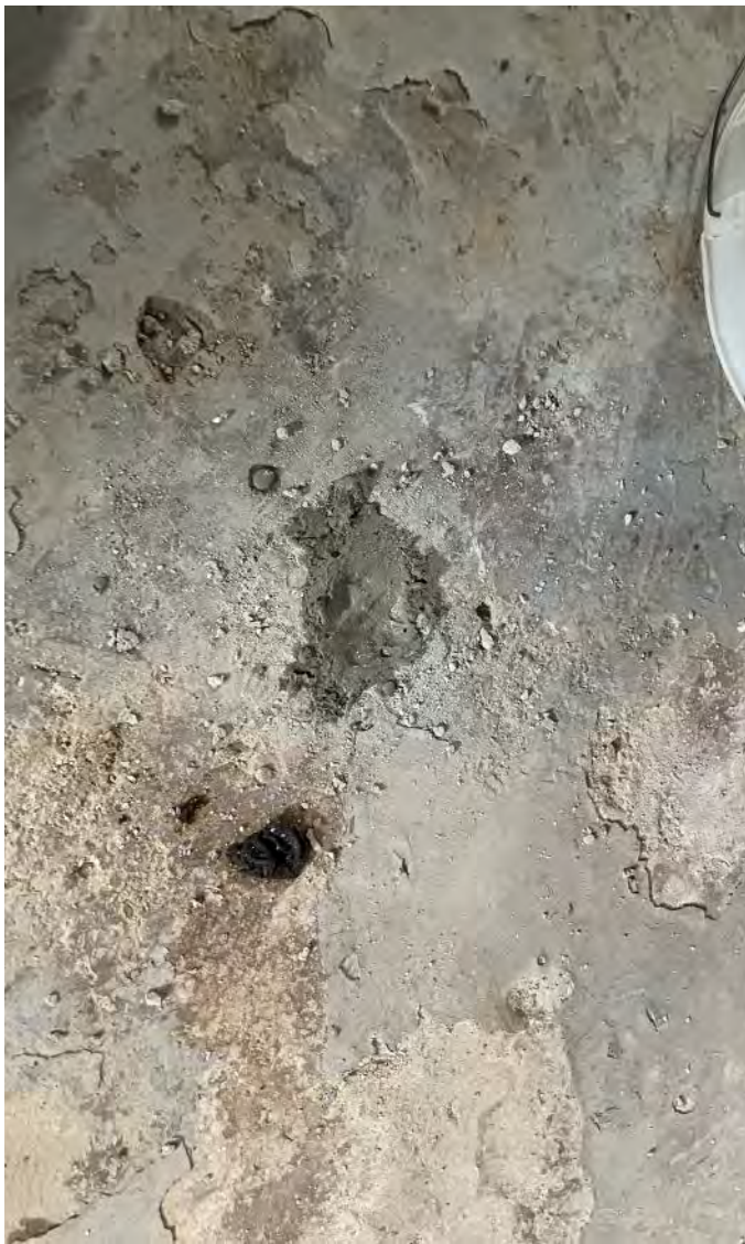
Photo 3: Temporary cement seal installed over the sample point. Photograph taken on June 9, 2023.
