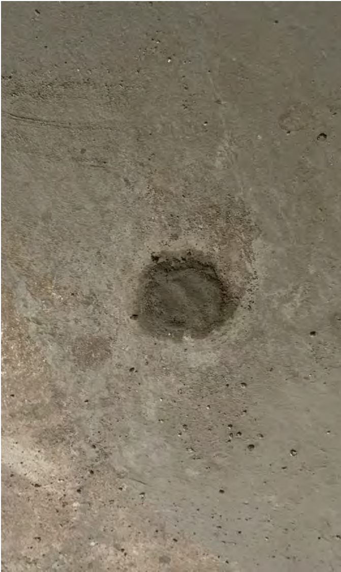
Photo 7: Abandonment of sample point on west side of basement. Photograph taken on February 16, 2024.
