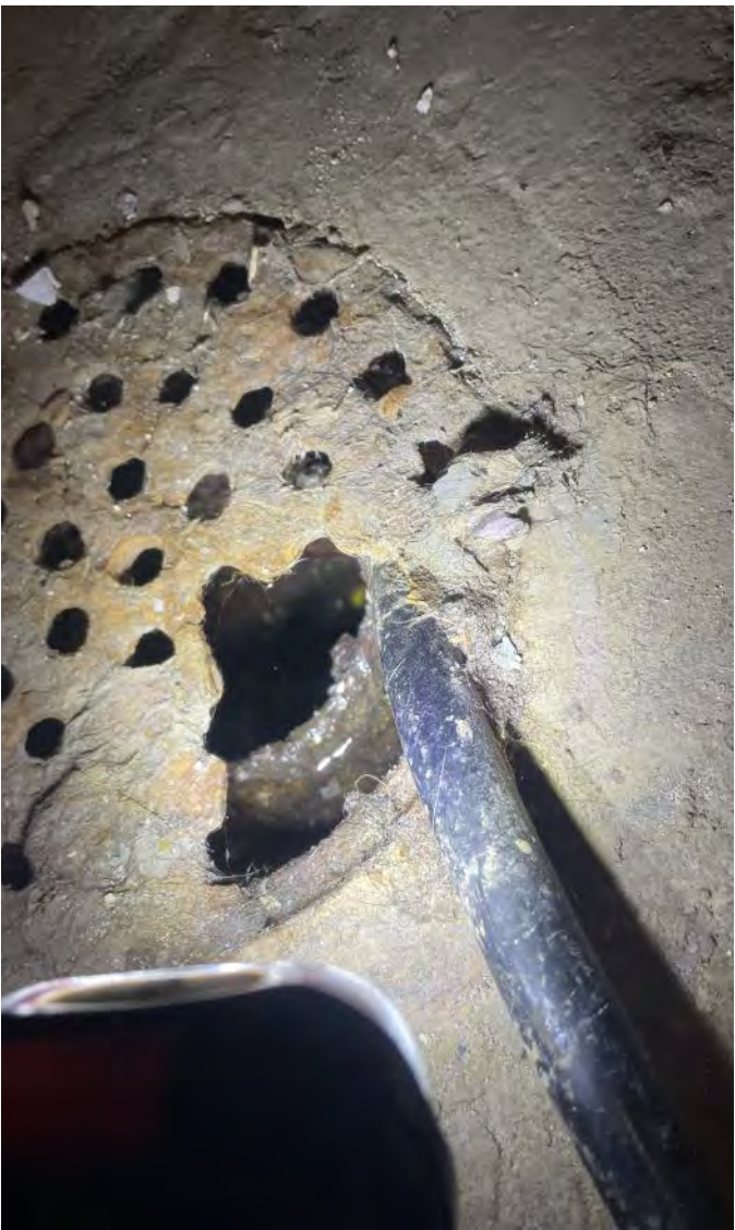
Photo 2: Floor drain within basement. Photograph taken on May 19, 2023.
