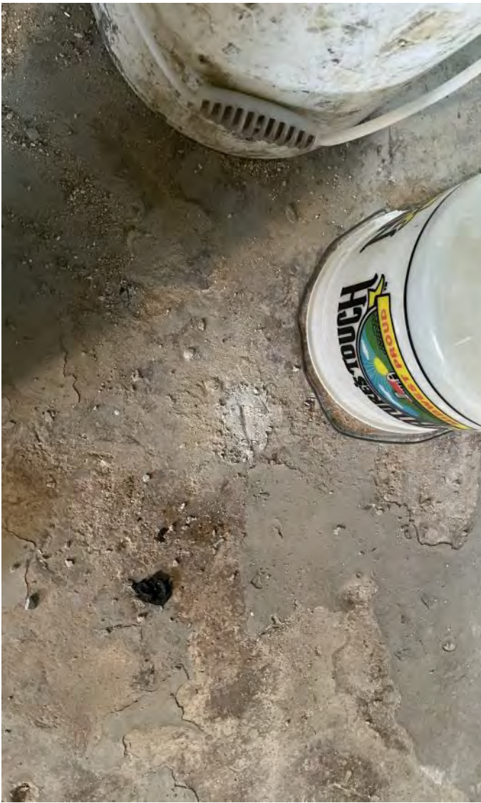
Photo 4: Sub-slab sample point abandoned on April 22, 2024.
