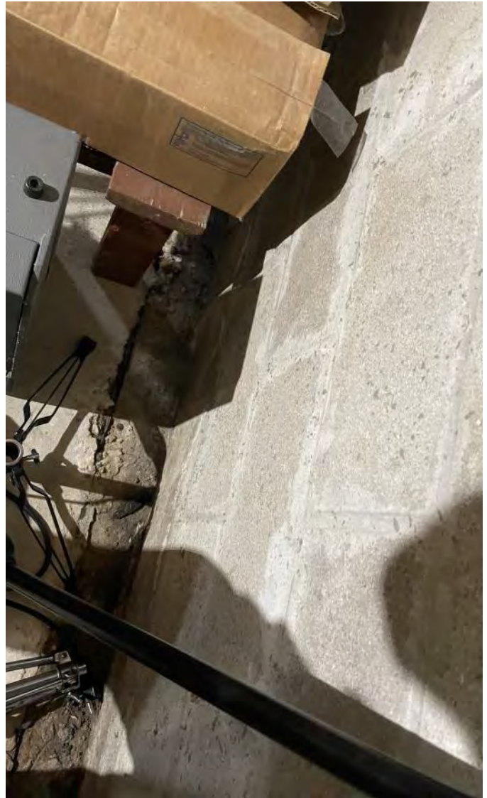
Photo 4: Perimeter joint around the exterior walls of the basement. Photograph taken on May 22, 2023.
