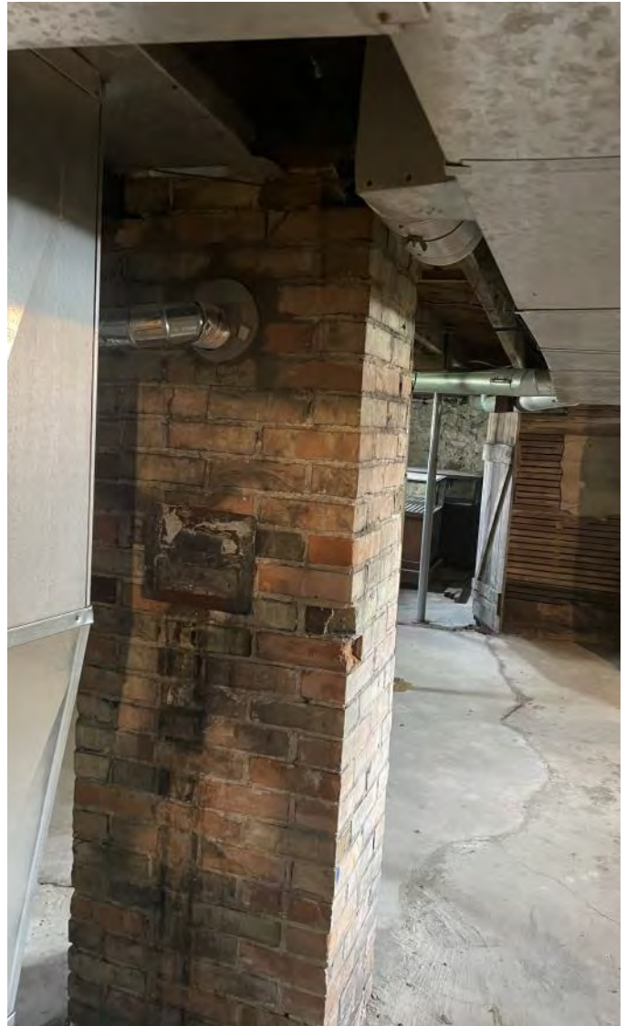
Photo 2: Brick column located within the central portion of the basement. Photograph taken on May 19, 2023.
