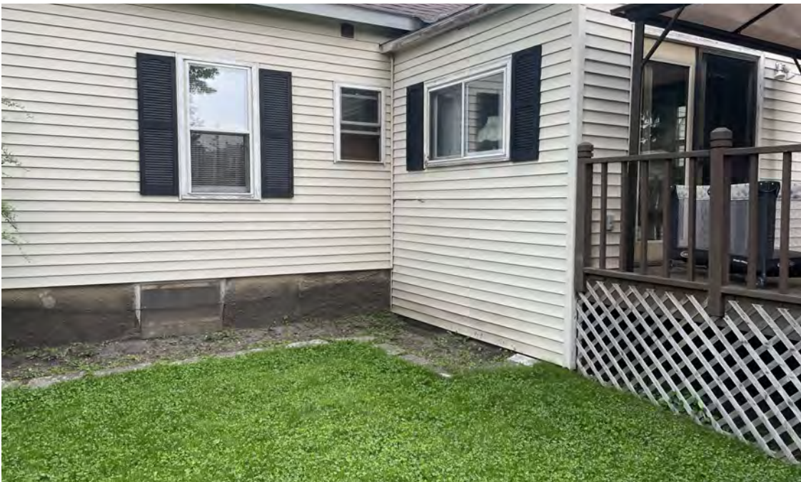
Photo 2: East side of residential home. View to the northwest; photograph taken on May 19, 2023.
