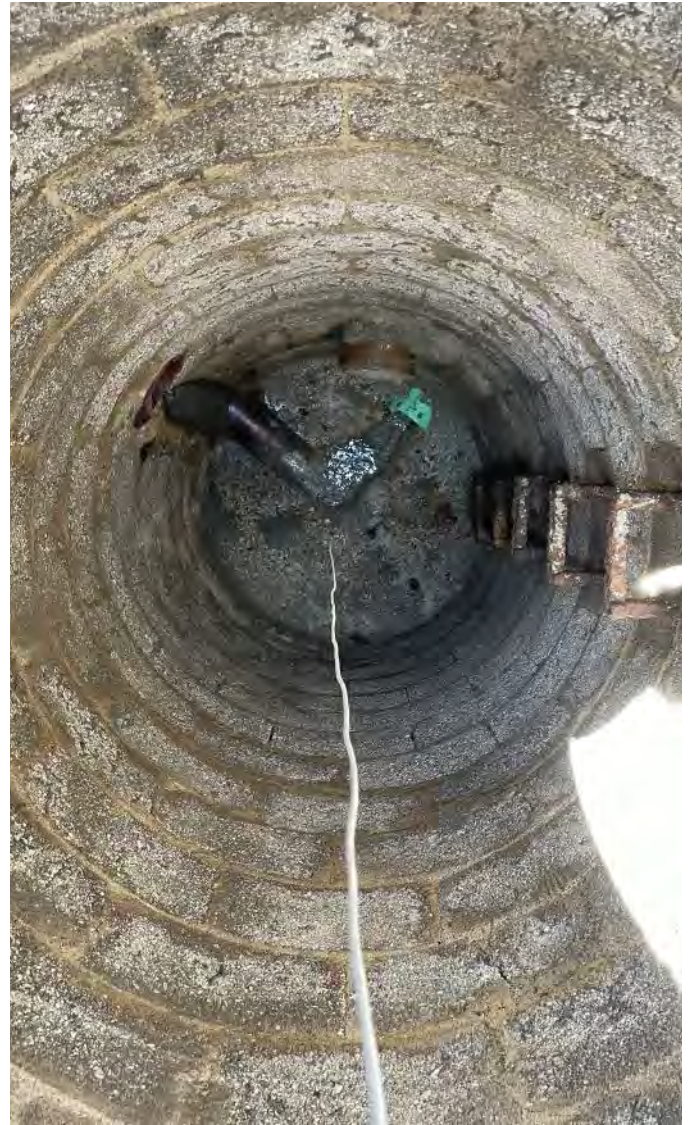
Photo 2: Sanitary sewer manhole sampler placement within the northern most manhole (105). Photograph taken on June 9, 2023.
