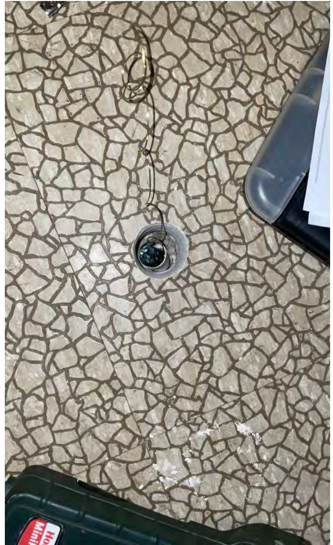
Photo 2: Installation of aluminum pipe into the drilling hole. Installation of passive sampler within the aluminum pipe. Photograph taken on June 12, 2023.
