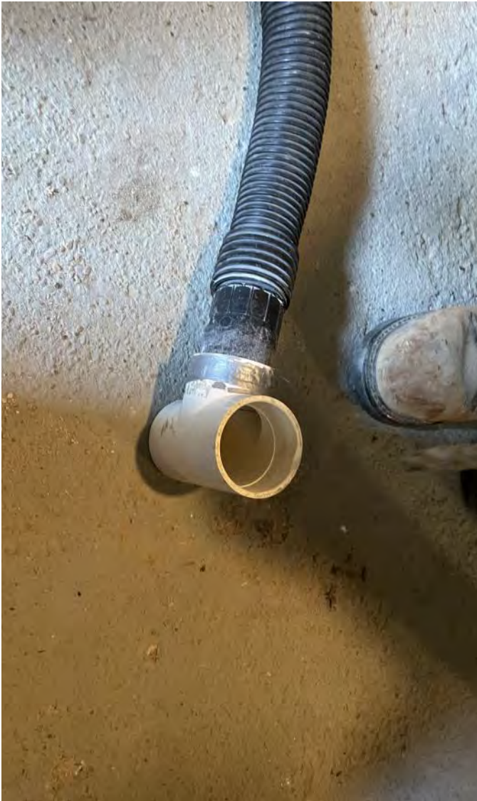
Photo 3: T-fitting installed on a shop vacuum used during drilling. Photograph taken on June 9, 2023.
