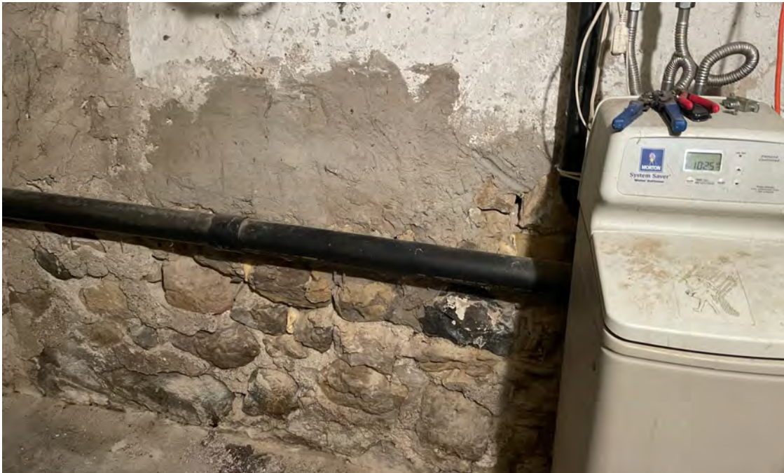
Photo 3: Stone wall with basement. Photograph taken on May 19, 2023.
