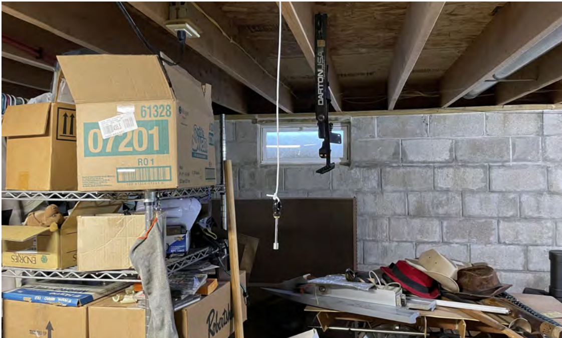
Photo 1: Indoor air sample located on the westside of the basement. Photograph taken on June 12, 2023.
