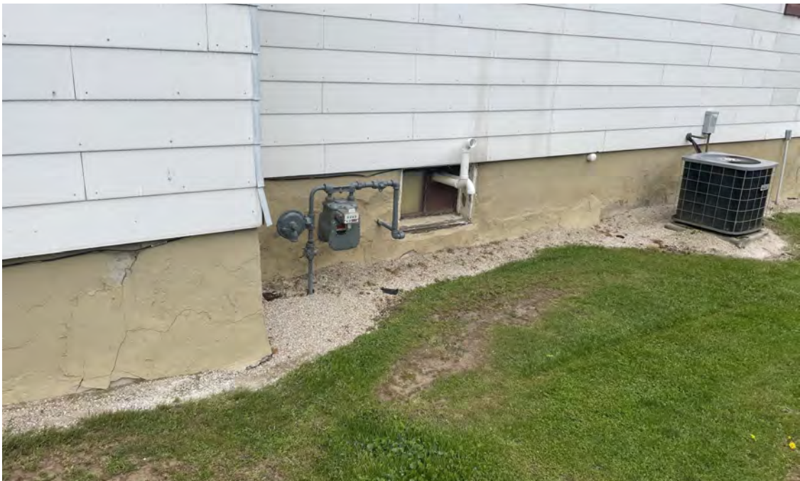
Photo 2: West side of home. View to the southeast; photograph taken on May 19, 2023.
