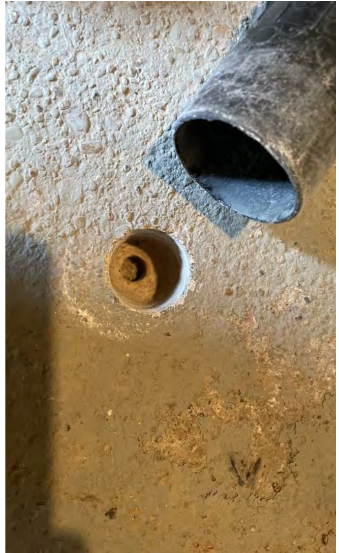
Photo 2: 5/8" diameter hole drilled approximately 4 to 6" into the base material. Photograph taken on June 9, 2023.
