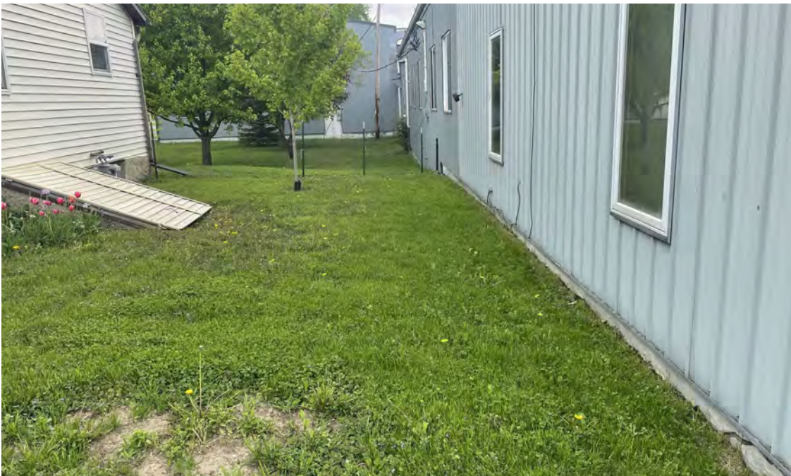
Photo 2: South side of residential home. View to the east; photograph taken on May 19, 2023.
