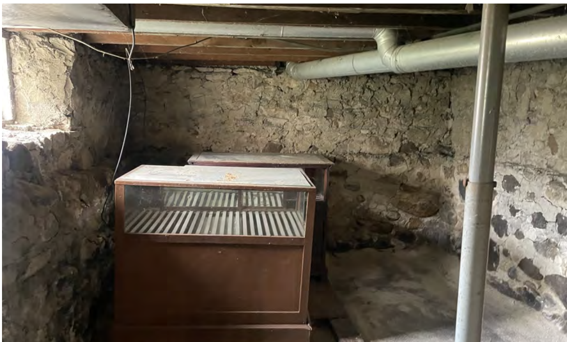
Photo 3: Stone wall located on the north portion of the home. Photograph taken on May 19, 2023.
