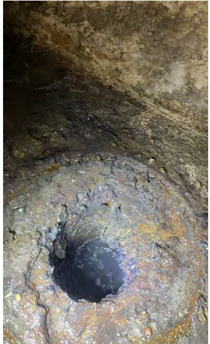
Photo 2: Floor drain located within the basement. Photograph taken on May 19, 2023.
