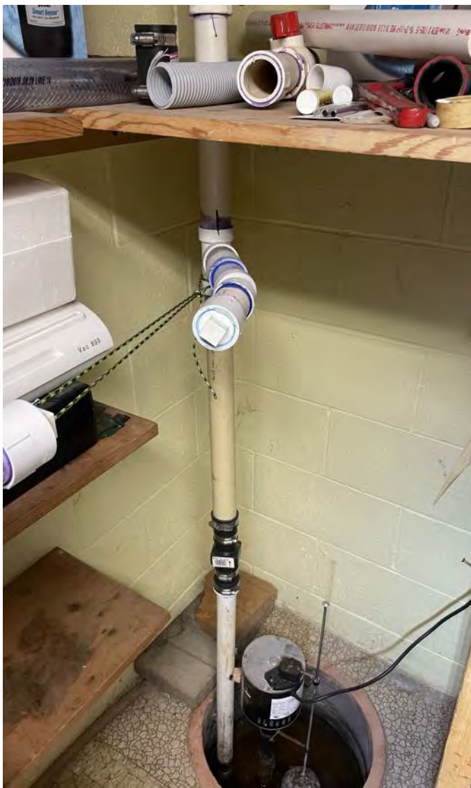
Photo 1: Basement sump within northeast corner of basement. Photograph taken on May 19, 2023.
