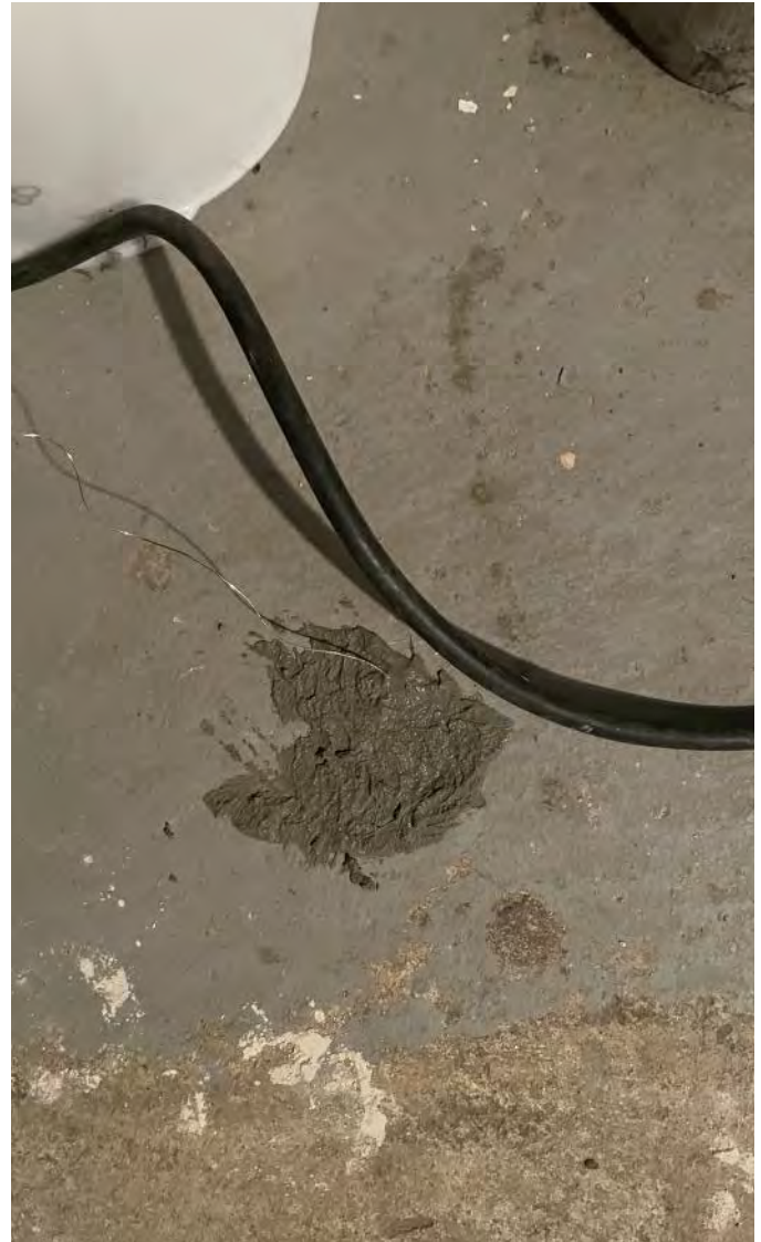
Photo 6: Temporary cement seal installed over the sample point located on the west side of the basement. Photograph taken on June 12, 2023.
