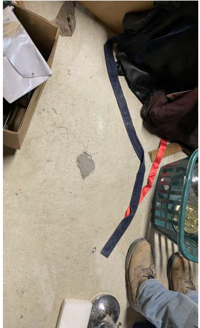
Photo 4: Temporary cement seal installed over the sample point. Photograph taken on June 12, 2023.
