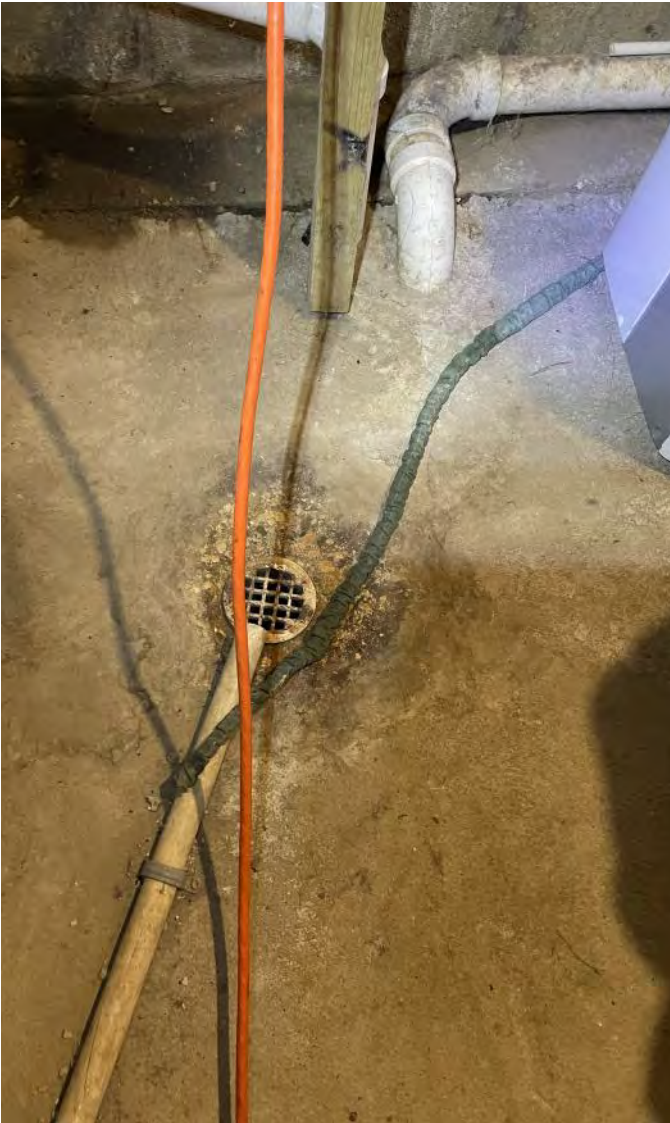
Photo 3: Floor drain located on the east side of the basement. Photograph taken on May 22, 2023.
