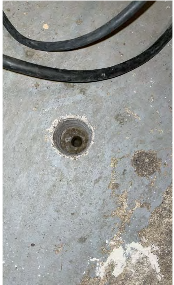
Photo 2: 1/5" diameter hole drilled through the concrete floor slab and the 5/8" diameter hole drilled approximately 4 to 6 inches into the base material. Location on the west side of the basement. Photograph taken on June 12, 2023.
