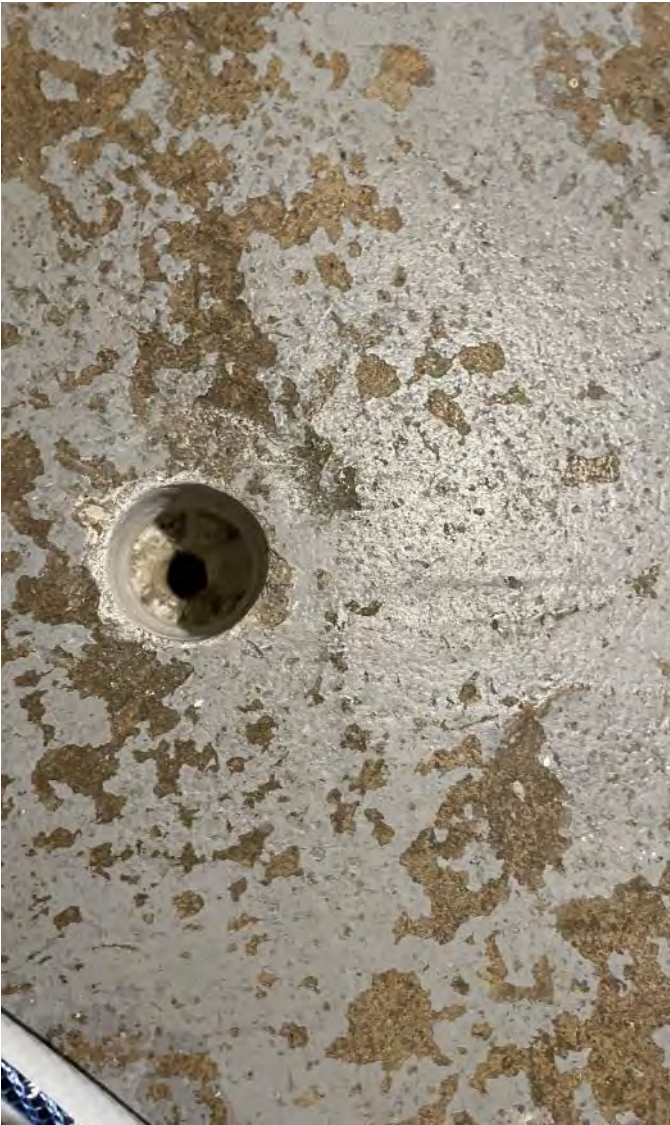
Photo 1: 1/5" diameter hole drilled through the concrete floor slab and the 5/8" diameter hole drilled approximately 4 to 6 inches into the base material. Location near floor crack. Photograph taken on June 12, 2023.
