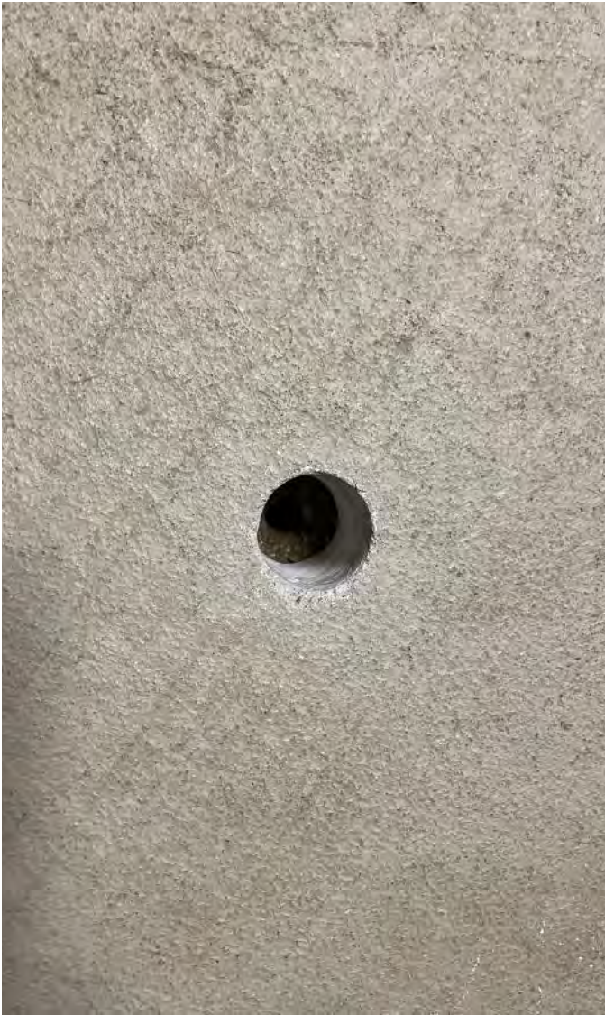
Photo 1: 1 1/2" diameter hole drilled through the concrete floor slab and the 5/8" diameter hole drilling approximately 4 to 6" into the base material. Photograph taken on June 12, 2023.
