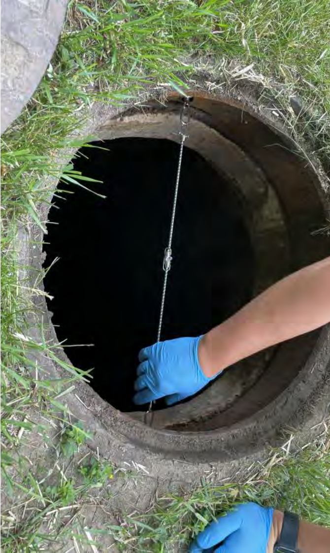
Photo 5: Sanitary sewer manhole sampler placement within the southern most manhole (103) using magnets and bungee cords. Photograph taken on June 9, 2023.
