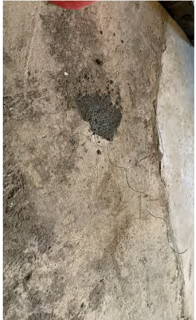
Photo 4: Temporary cement seal installed over sampling point with retrieval wire present out side of the hole. Photograph taken on June 9, 2023.
