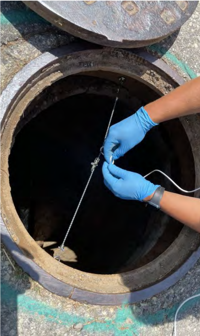
Photo 3: Sanitary sewer manhole sampler placement within the middle manhole (104) using magnets and bungee cords. Photograph taken on June 9, 2023.
