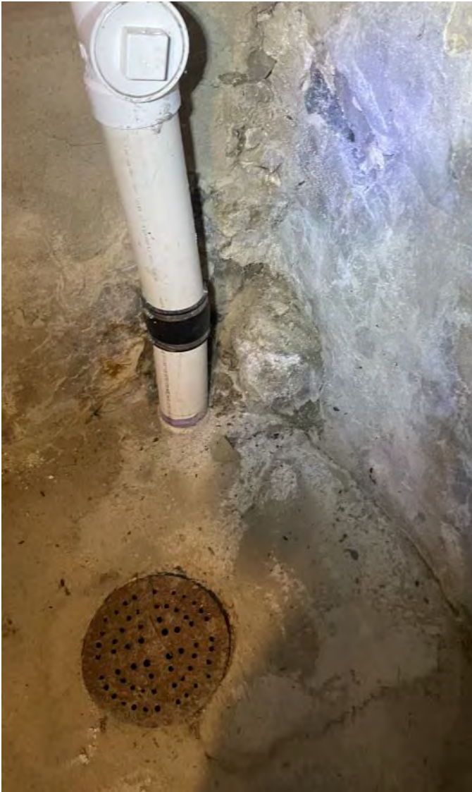
Photo 3: Floor drain located on the south side of the basement. Photograph taken on May 19, 2023.
