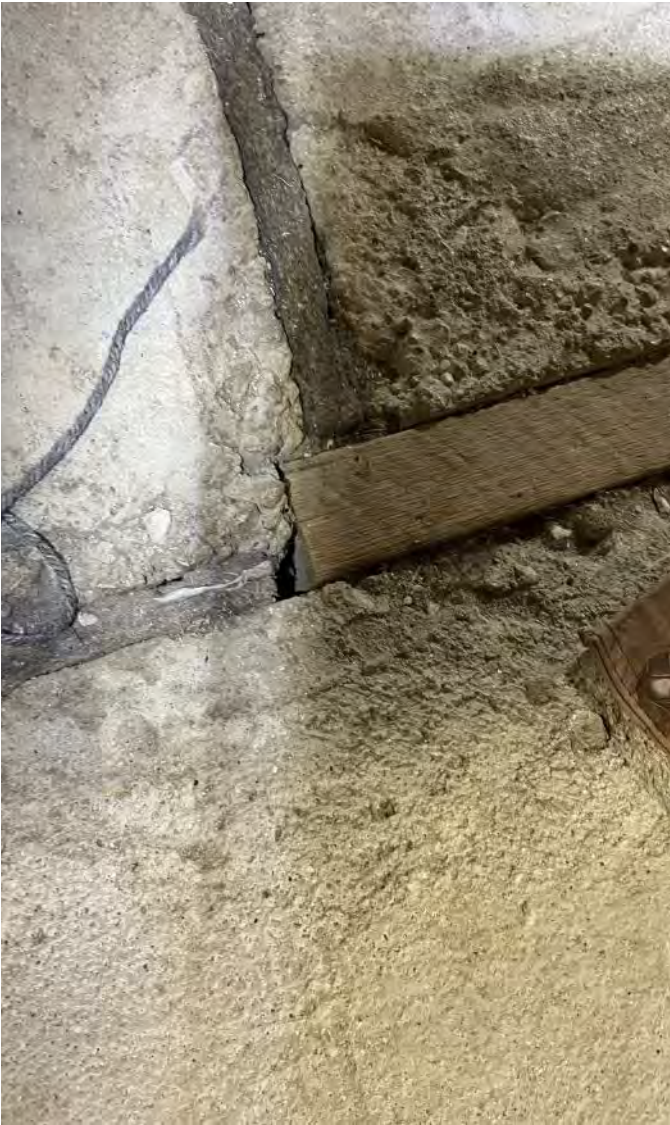
Photo 5: Wooden forms left in place when the basement floor was poured. Photograph taken on May 22, 2023.
