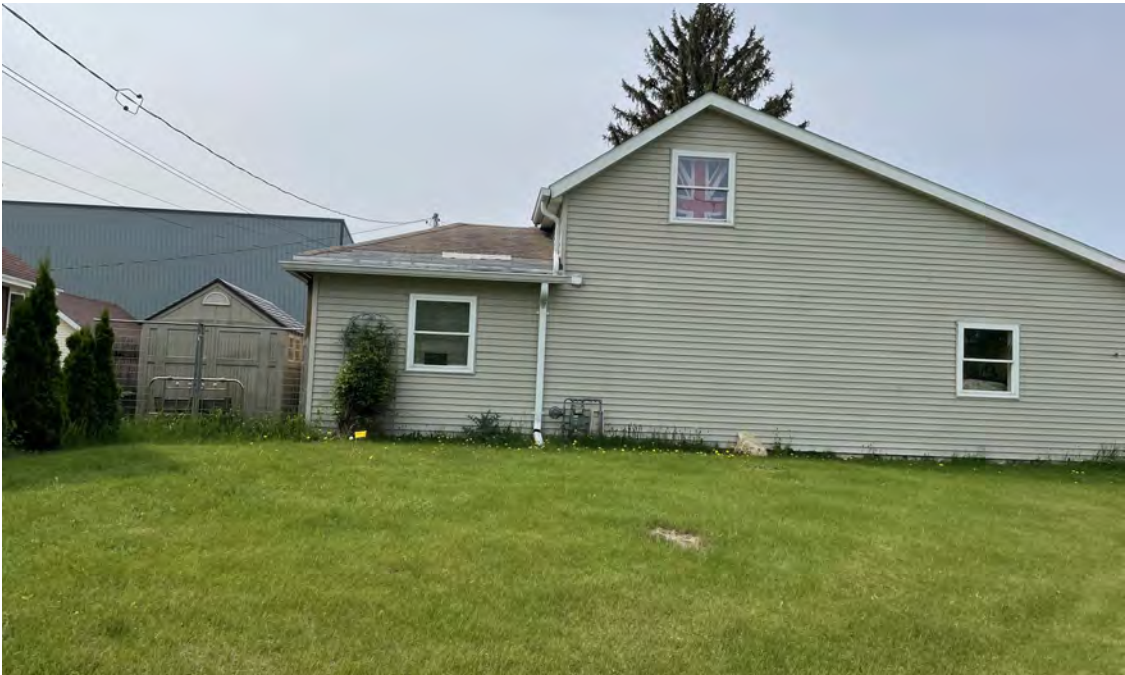
Photo 2: North side of home. Photograph taken on May 22, 2023.
