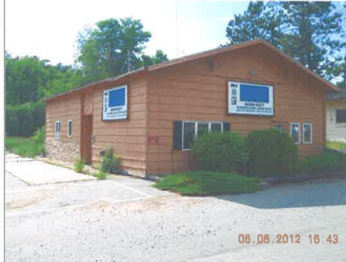
Title: Looking northwest at the former Smiths Union 76 Station building.
