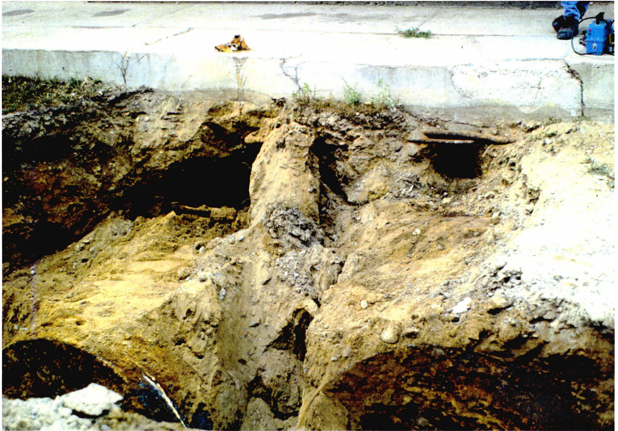
TANKS LOCATED ADJACENT TO CONCRETE SLAB
