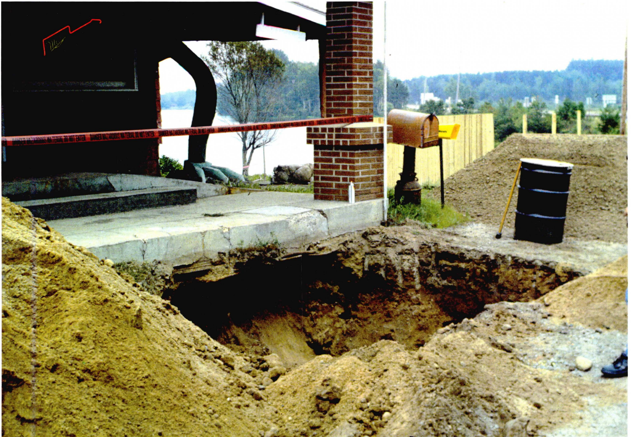
TANK EXCAVATION AND FOUR SEASONS TAVERN
