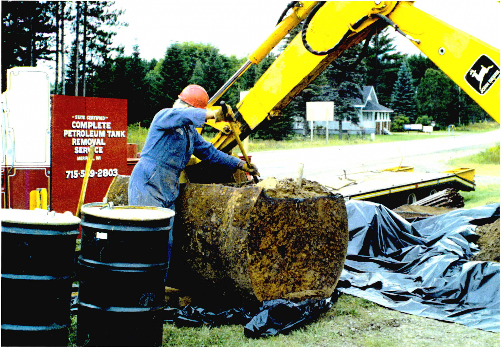
REMOVING SAND FROM TANK
