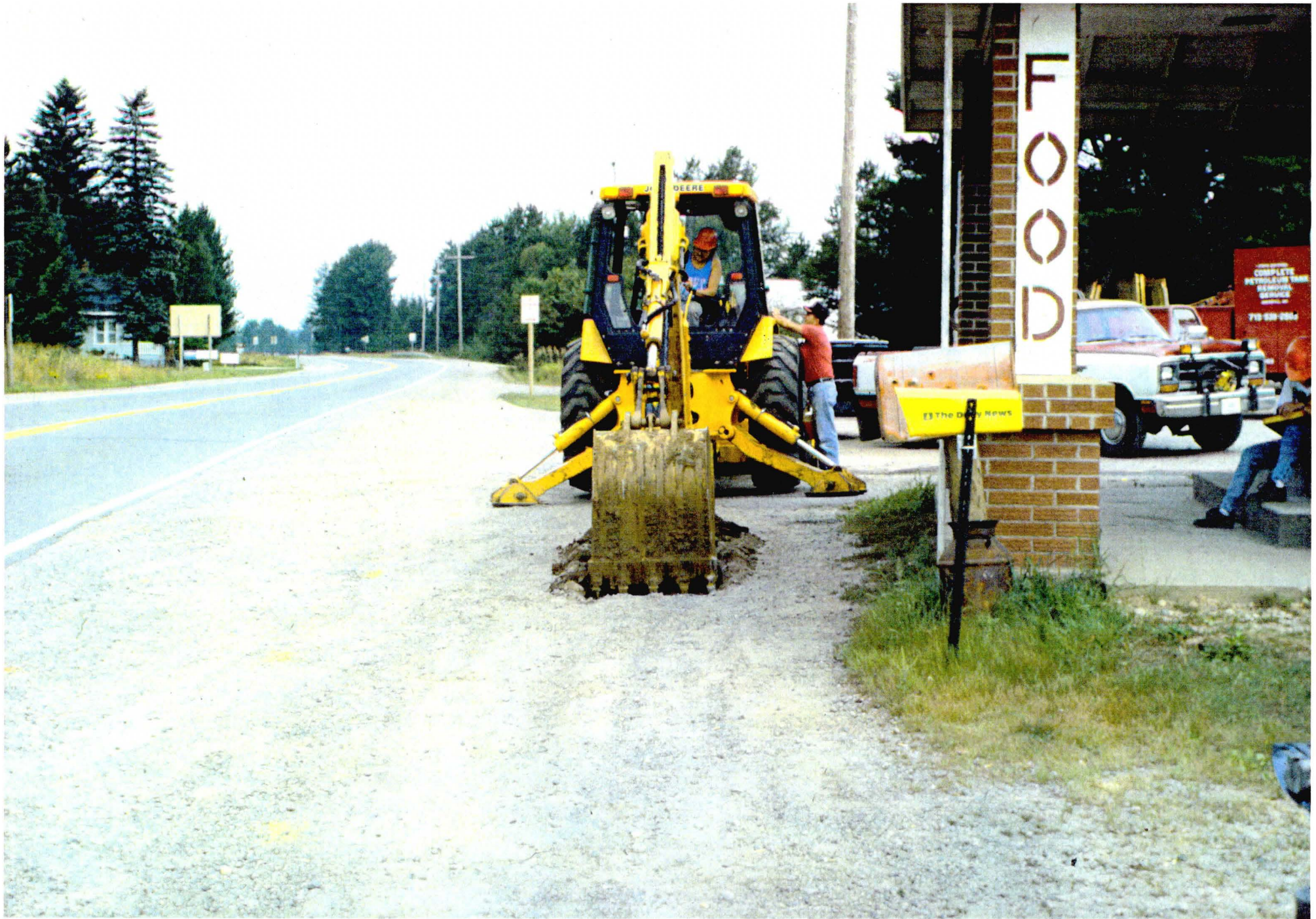
SEARCHING FOR TANKS WITH BACKHOE
