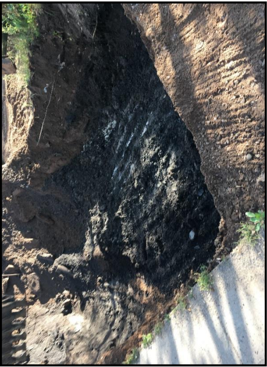
Southwest corner to 4 feet - complete
