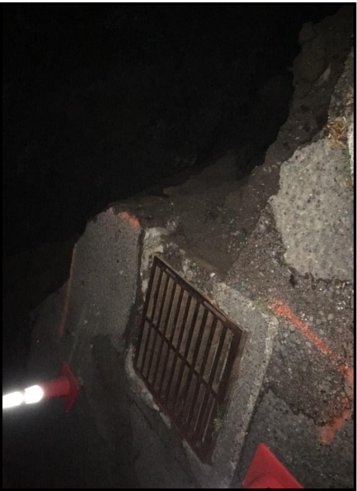
Excavation adjacent to catch basin in northwest corner
