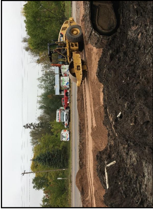
Compacting backfill
