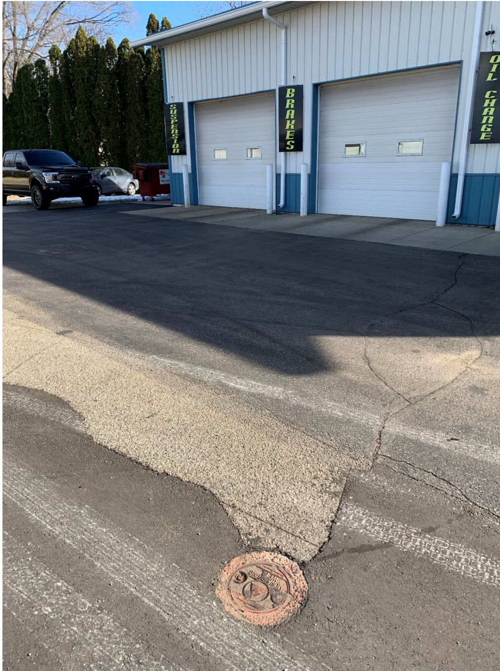
Asphalt cap to be maintained. MW2 in foreground, Jim's Service building in background. Photo taken November 22, 2022.
