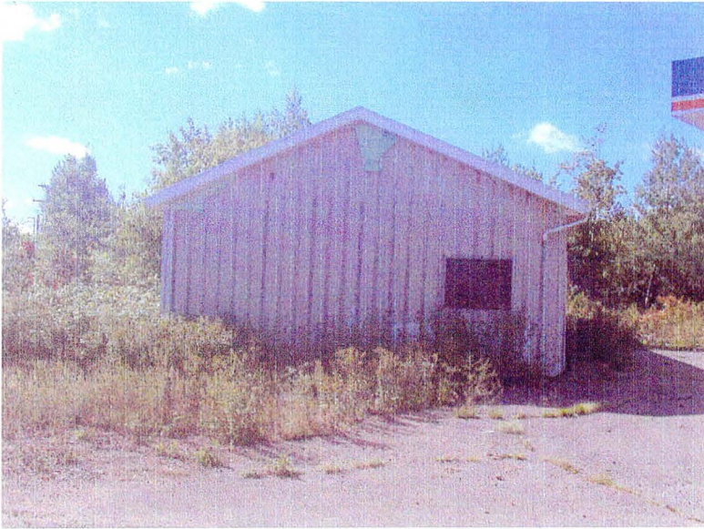
North side of building, looking south
