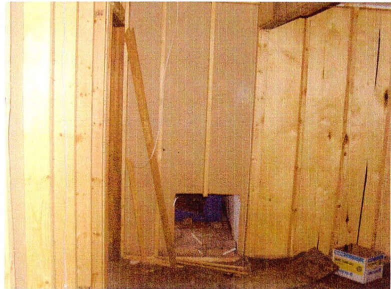
View of possible heater vent hole inside building
