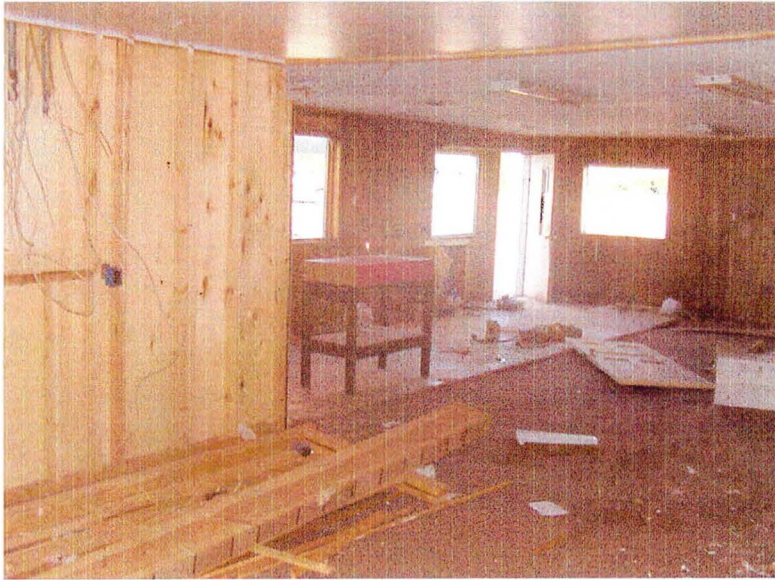
View of inside looking toward the northwest entrance
