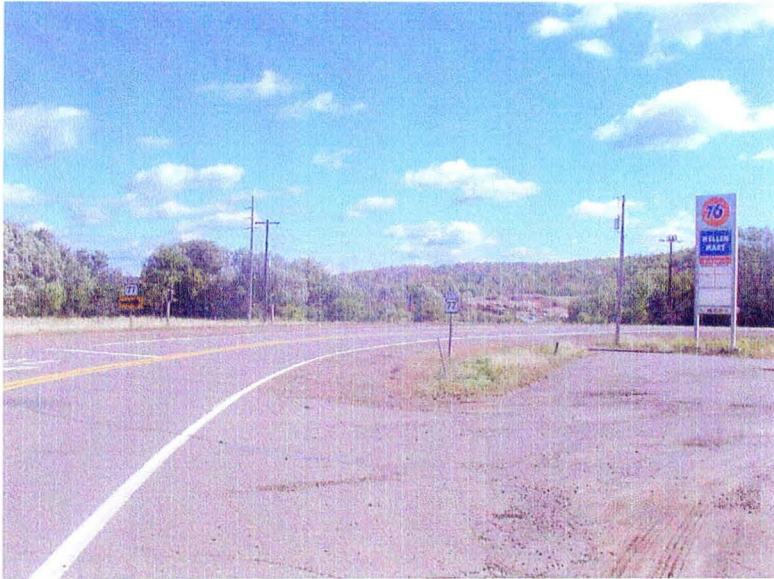
View along STH 77 looking along NE edge of property
