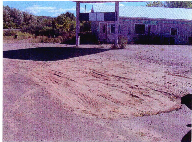
Fill area in former location of USTs
