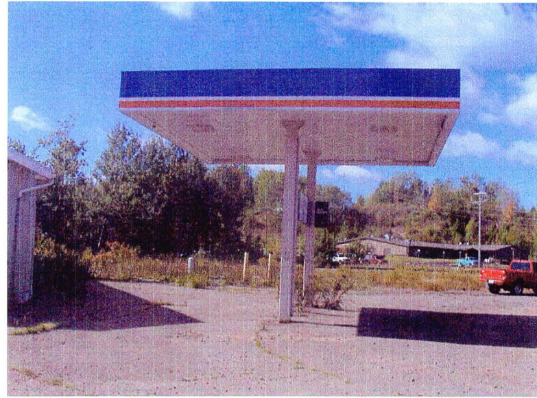
Remaining tank fueling area canopy, looking south
