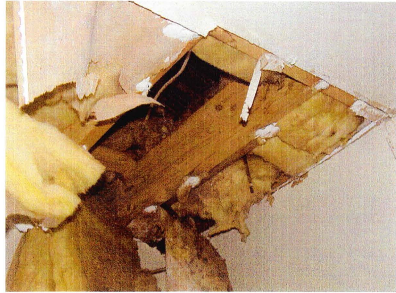
Fiberglass batt insulation inside cooler area
