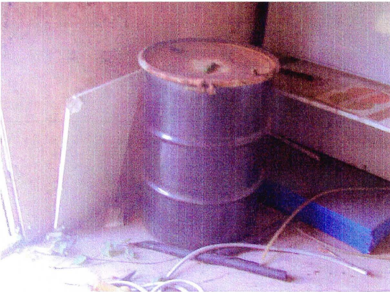
Empty 55-gallon drum inside southwest entrance to building
