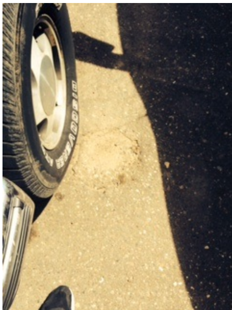
East side near excavation MW patch
