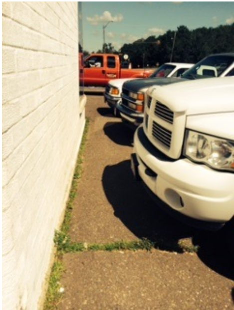
North view adjacent to building
