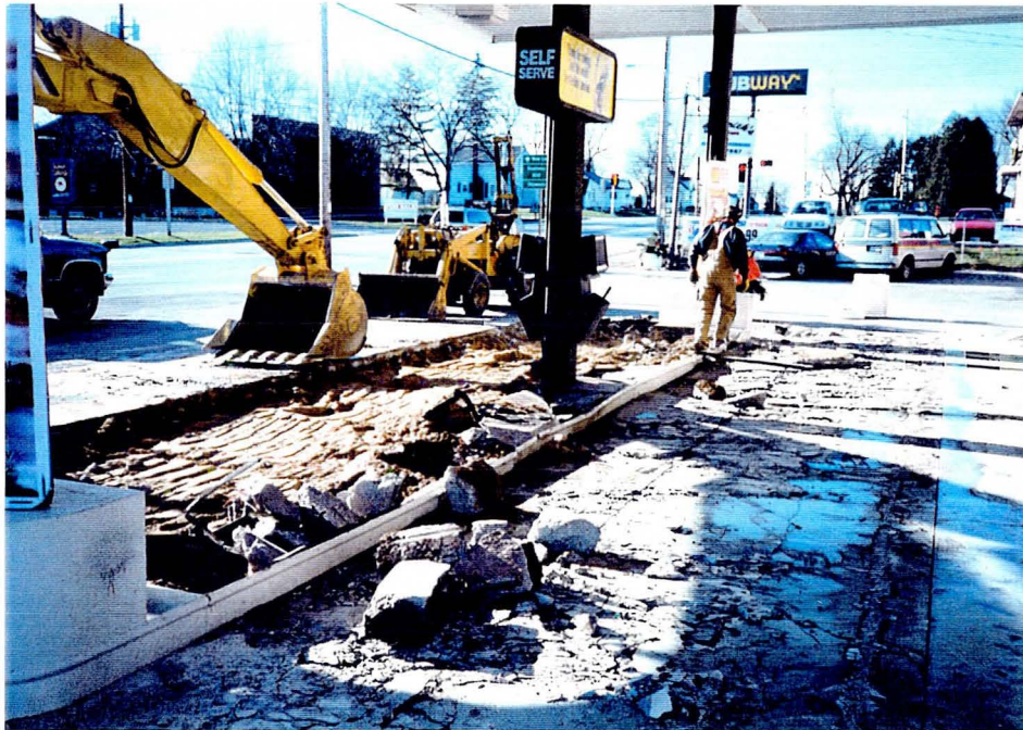
PHOTO 3 View of the dispenser island to the south of the building.
