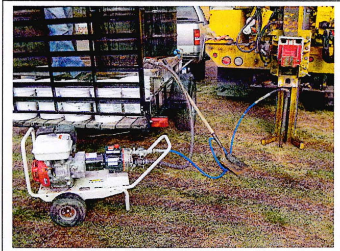
Facing: Photo 5 View of: RegenOx™ Injection point. November Event
