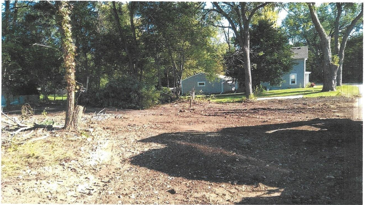
Looking northeast at Excavation Area D
