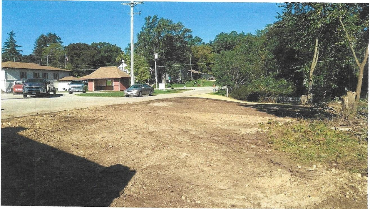
Looking northwest at Excavation Area A
