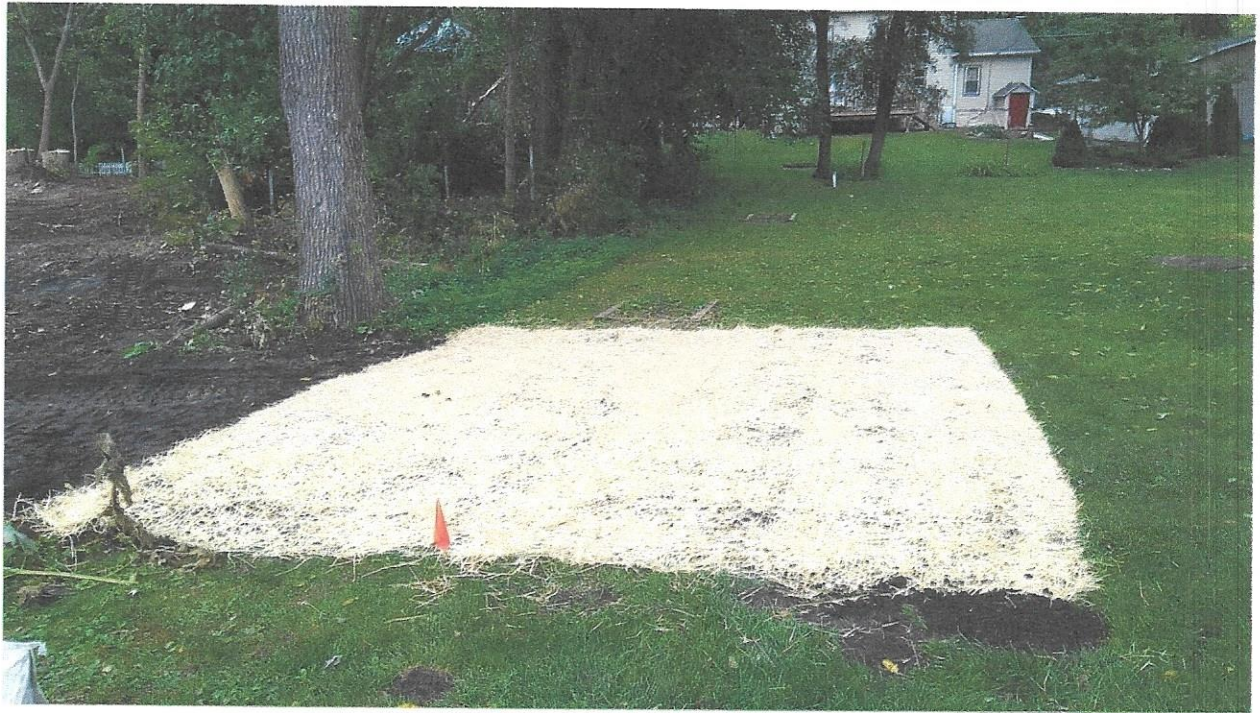
Looking northwest at Excavation Area C
