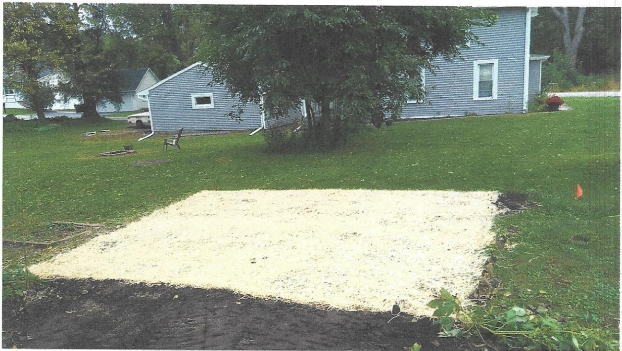
Looking northeast at Excavation Area C
