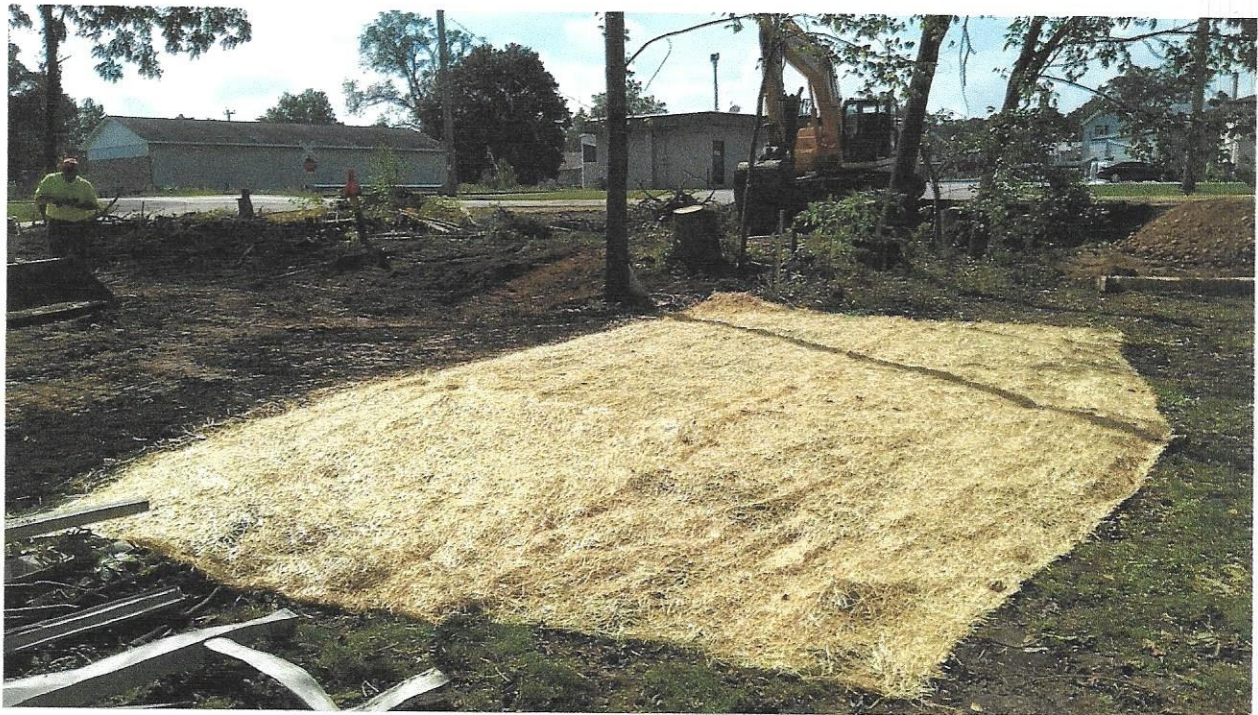
Looking south at Excavation Area B
