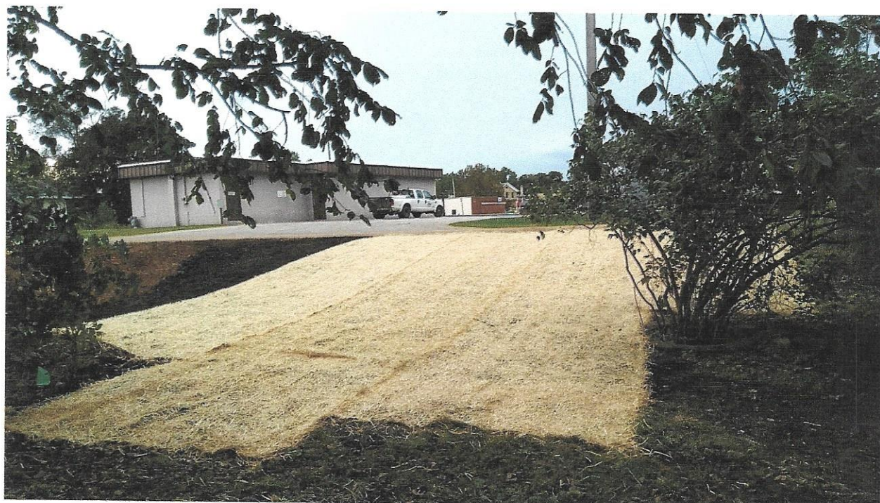
Looking south at Excavation Area A
