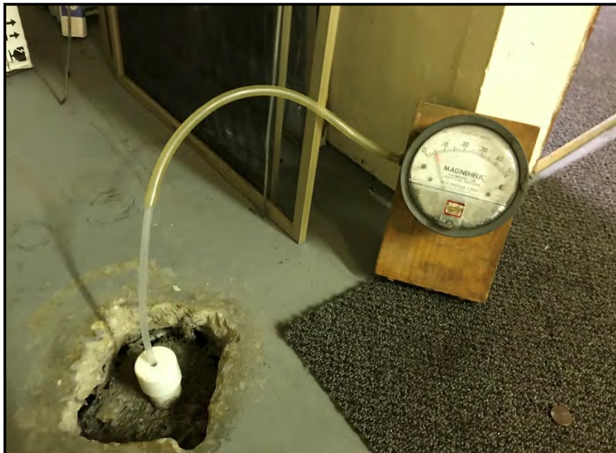
Vacuum at TW900- 0.05" water
