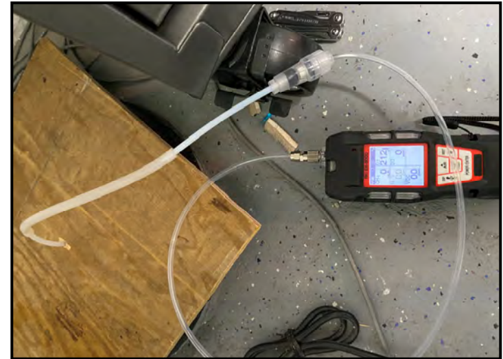
Purging sump pit 4/14/22
