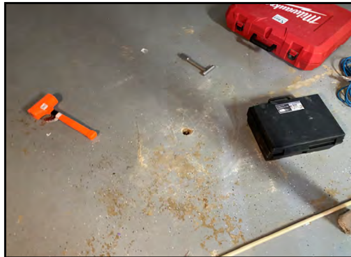
Vapor pin installed - 716 Lincoln Street
