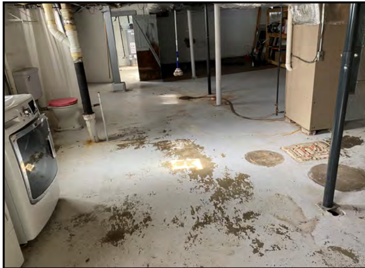
866 Mather Street, basement
