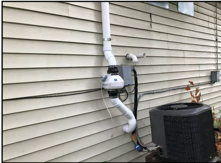
Fan location - near northwest corner of building
