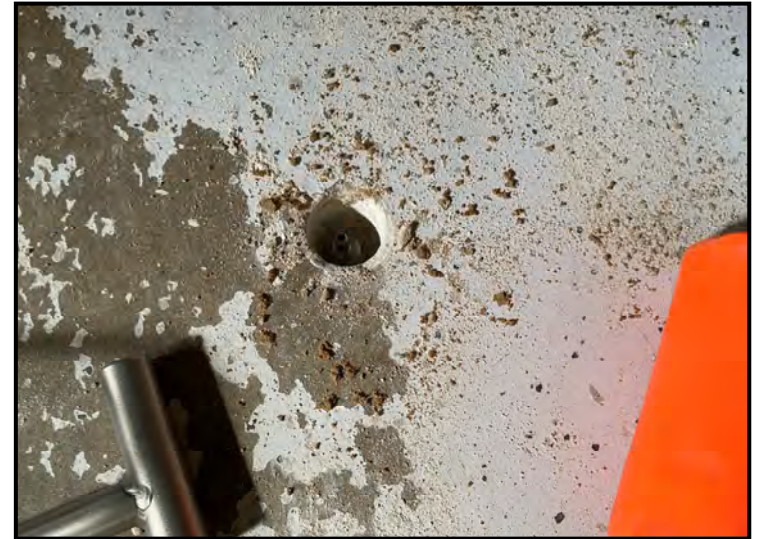
Vapor pin installed
