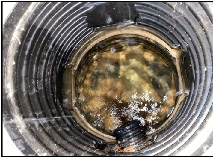
Interior of sump pit
