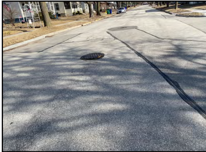
Downgradient manhole near intersection of Lincoln Street and James Street
