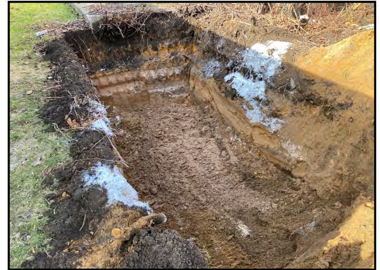
Completed excavation, view to south
