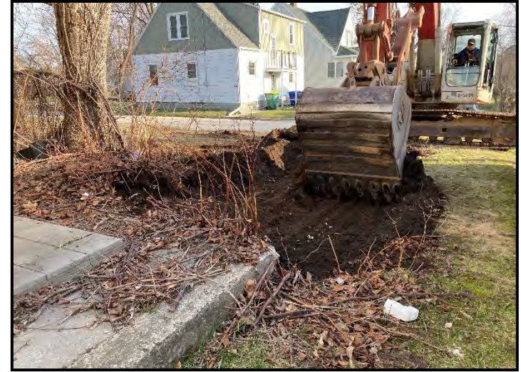
Excavating soil - large tree to west
