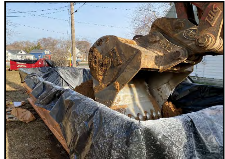
Loading roll-off boxes
