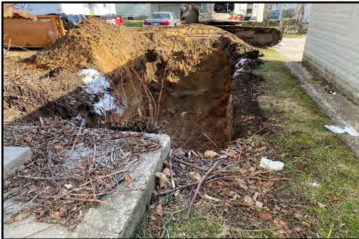
Completed excavation, view to north
