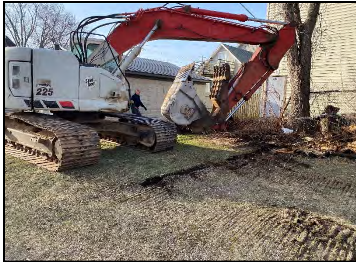
Removing topsoil
