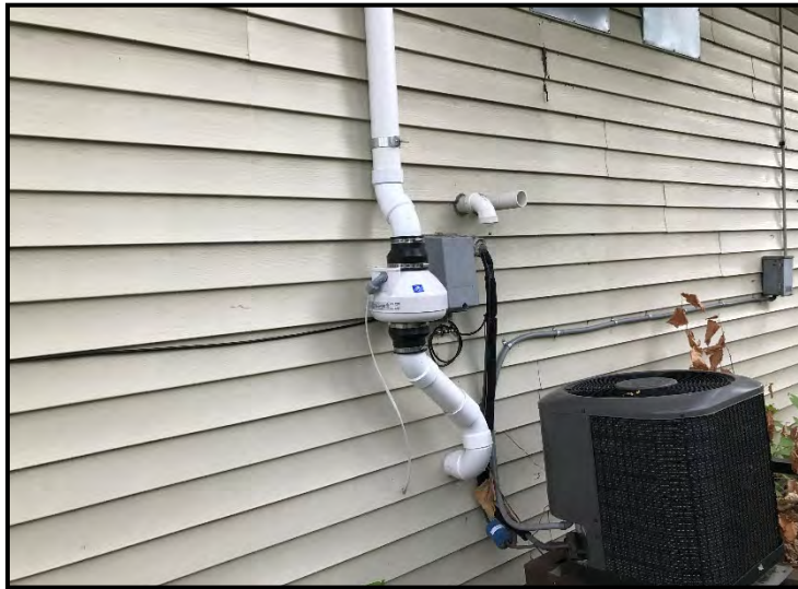
Fan location - near northwest corner of building
