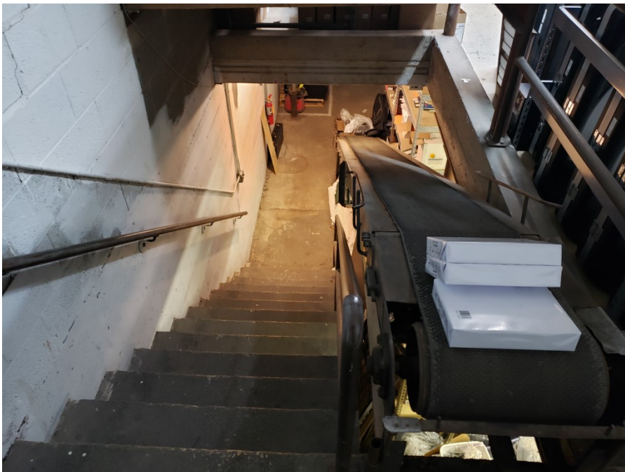
Photo 12: Stair opening to basement, Jim's Music (4/2/20; 12:39).
