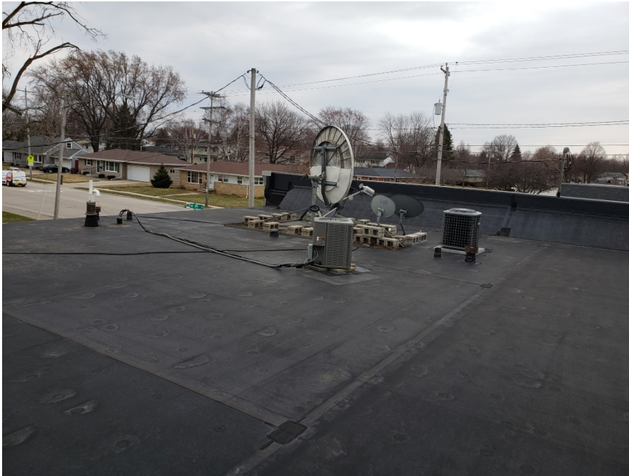
Photo 28: Roof of 1235 and 1239 units (4/3/20; 14:30).
