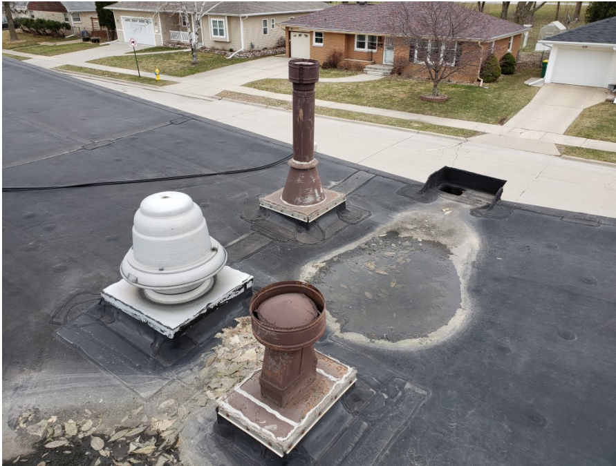
Photo 30: Bathroom fan vents (rusty) and basement exhaust fan (gray) at common wall between 1231 and 1219 units (4/3/20; 14:32).
