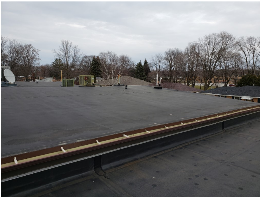
Photo 29: Roof of 1231 unit (4/3/20; 14:30).
