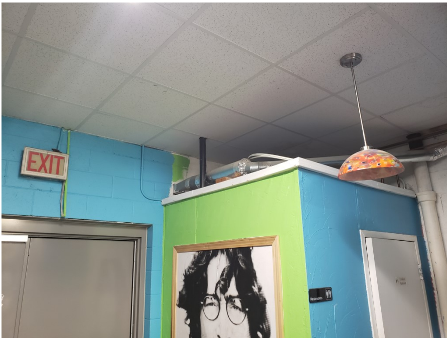
Photo 10: Plumbing vents (black 2-inch ABS and white 4-inch cast iron) at rear bathroom, Jim's music (4/2/20; 12:29).
