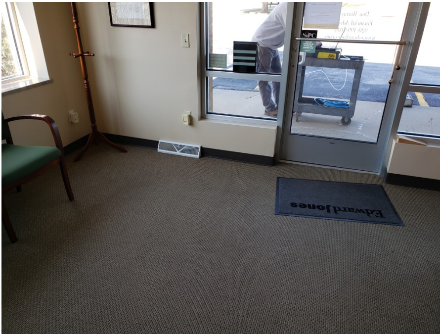
Photo 3: Edward Jones front reception area with floor register (4/2/20; 10:09).
