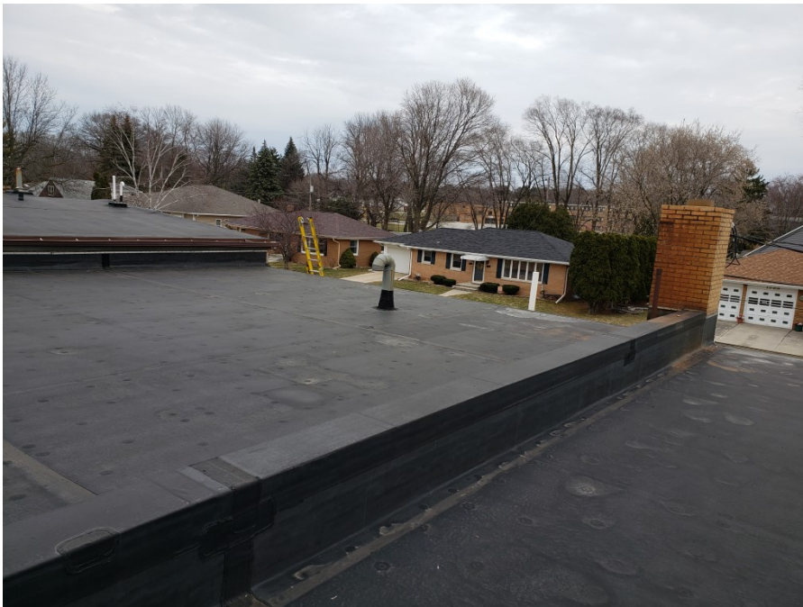
Photo 27: Roof of dry cleaner showing boiler room chimney and cleaning machine vent (galvanized pipe), (4/3/20; 14:30).
