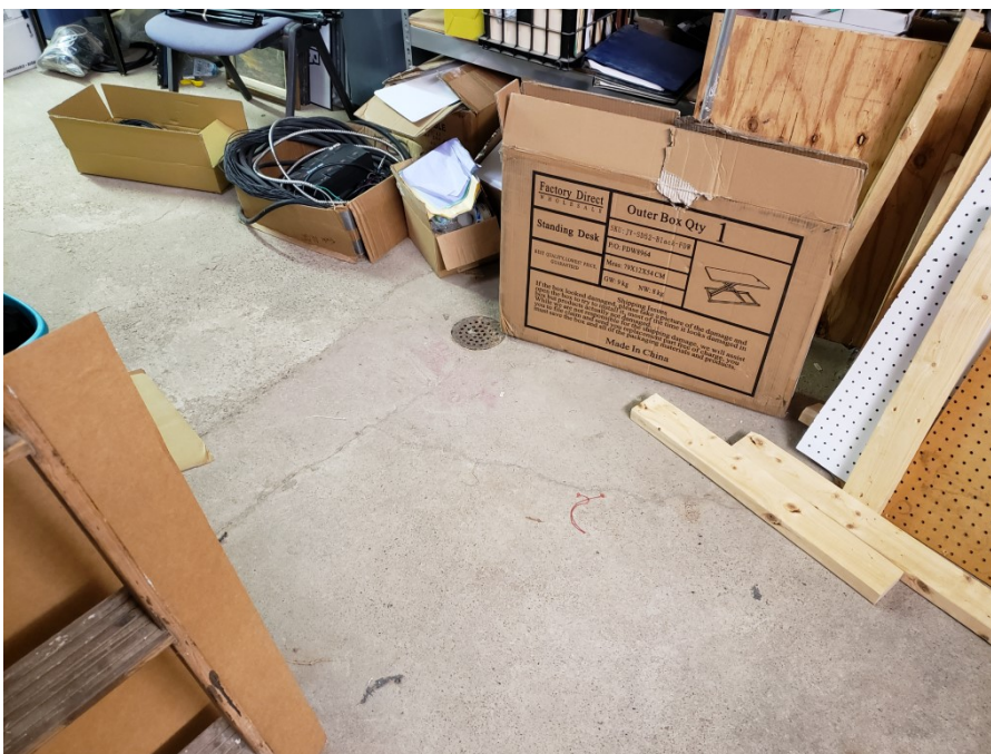
Photo 15: Floor drain in Jim's basement near stairwell (4/2/20; 13:01).
