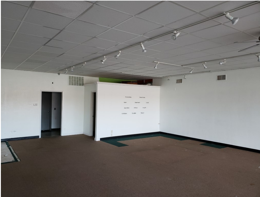
Photo 5: Former Williams Tae Kwon Do (unit 1235) back and south walls with HVAC vents near ceiling (4/2/20; 10:50).
