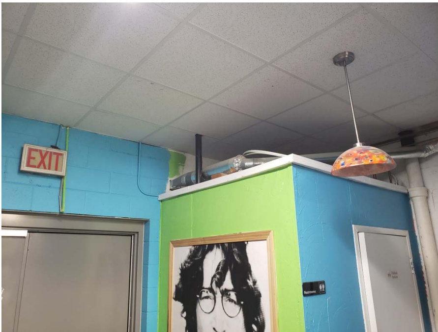
Photo 10: Plumbing vents (black 2" ABS and white 4" cast iron) at rear bathroom, Jim's music (4/2/20; 12:29).
