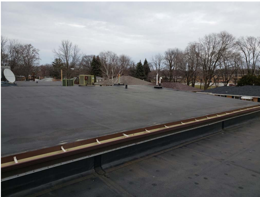
Photo 29: Roof of 1231 unit (4/3/20; 14:30).
