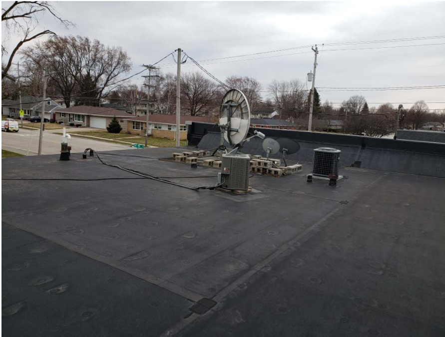
Photo 28: Roof of 1235 and 1239 units (4/3/20; 14:30).
