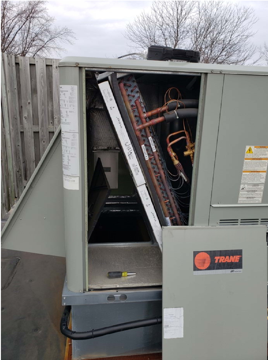
Photo 32: Roof-top HVAC unit at Jim's (unit 1219) showing damper for indoor return air (4/3/20: 14:45).
