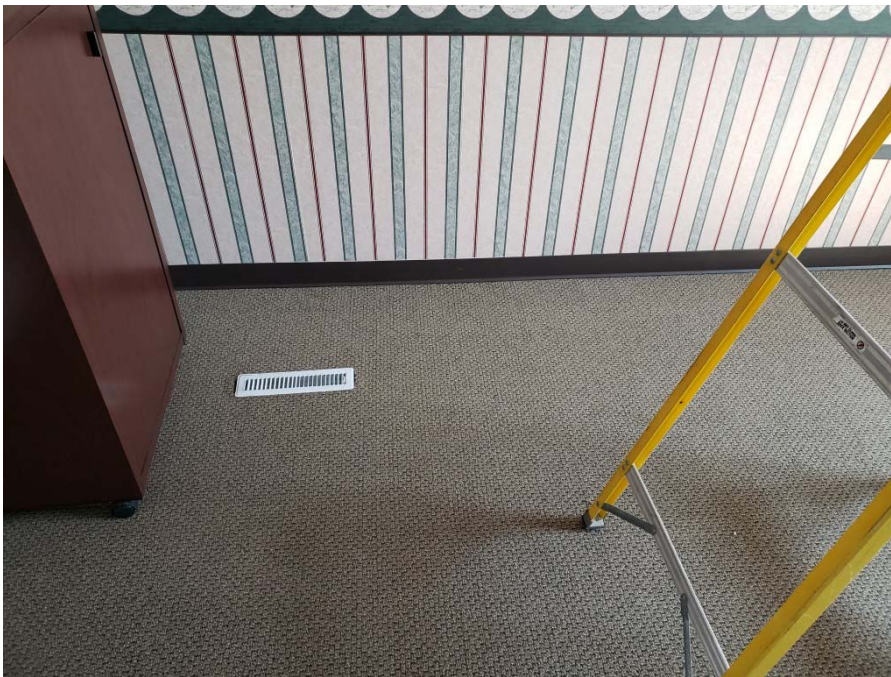
Photo 2: Edward Jones back office with floor register 4/2/20; 10:08).
