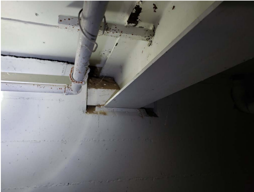
Photo 20: Beam pocket in south wall of Jim's annex basement 4/2/20; 13:53).
