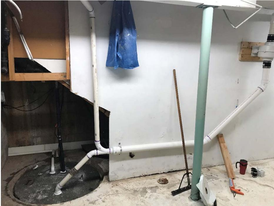
**Photo 10. Vacuum extraction points P7, west wall of north basement. Before and after sealing.**
