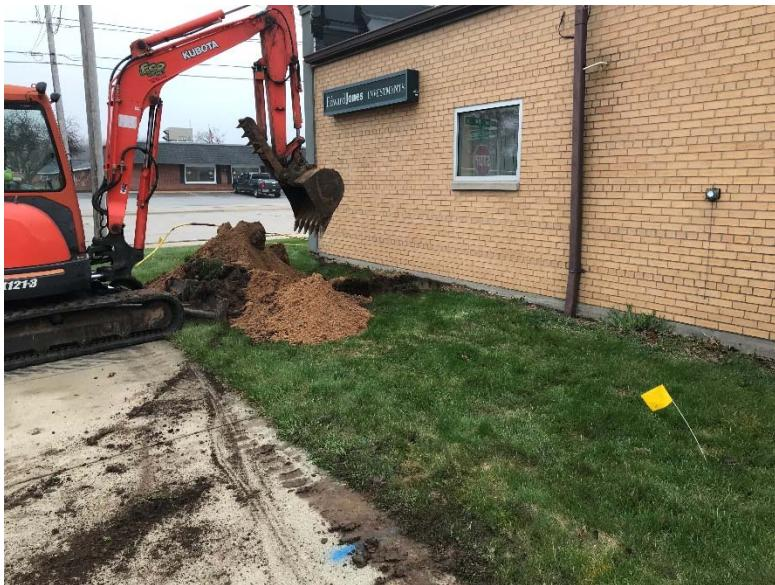
***Photo 2. Installation of East Wall Vapor Extraction Points***
