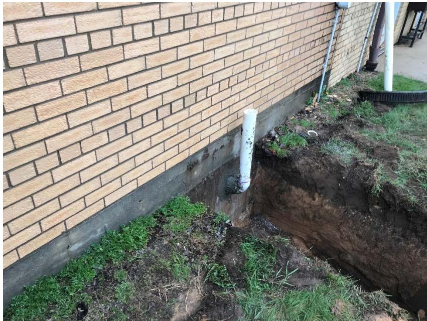
***Photo 4. East wall vapor extraction points.***
