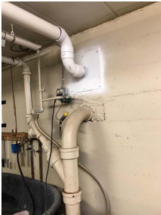
**Photo 12.** Vacuum extraction blower B2, north basement.
