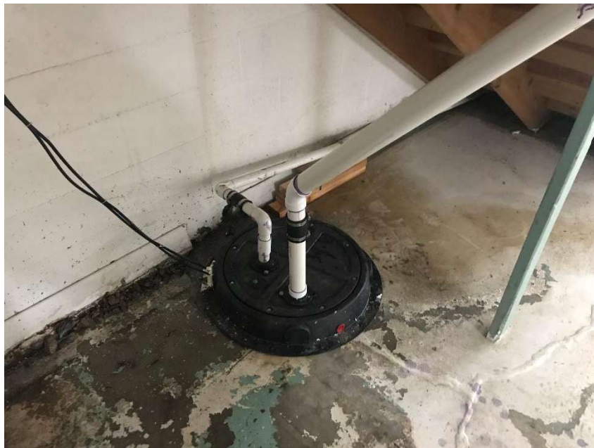
Photo 16. Sump S4, south basement.
