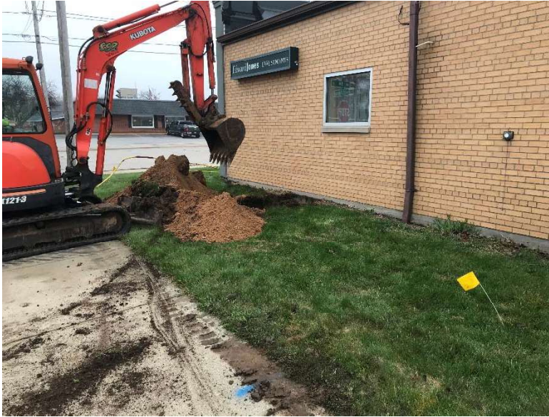
Photo 1. Installation of East Wall Vapor Extraction Points
