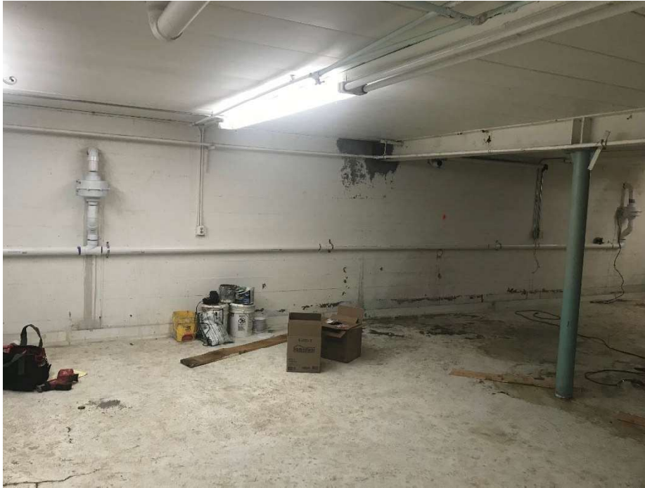
Photo 7. South basement vacuum blowers. Vacuum Blower B4 and B5.
