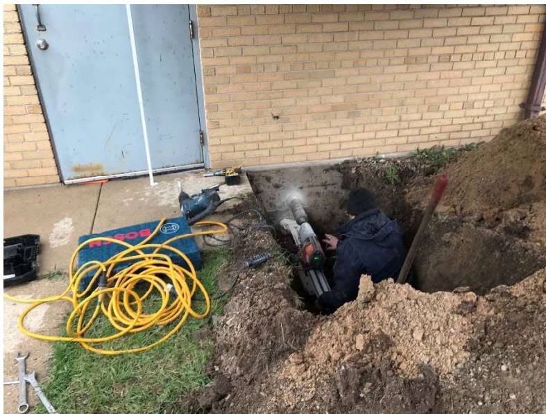
Photo 2. Installation of East Wall Vapor Extraction Points
