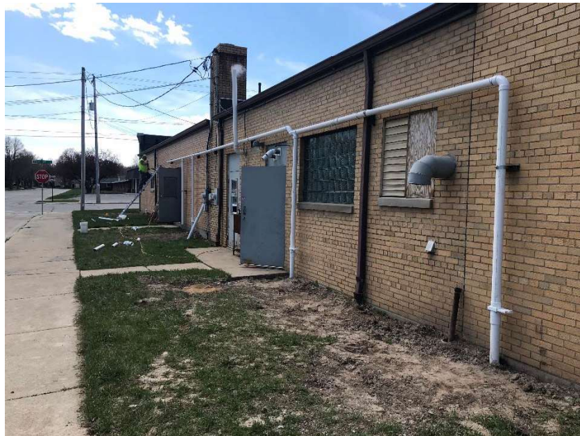
Photo 4. East wall vapor extraction points.
