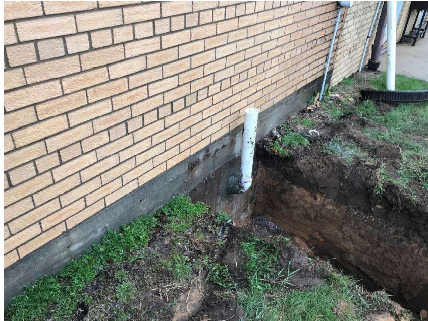
Photo 4. East wall vapor extraction points.
