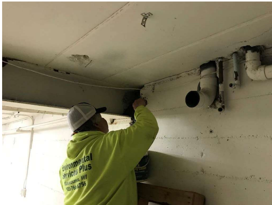
Photo 6. Sealing beam pocket in south basement.
