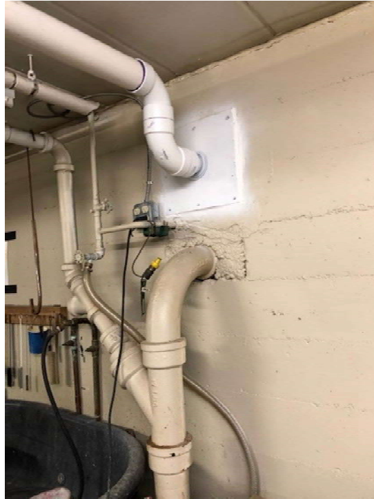
Photo 11. Vacuum extraction points P7, west wall of north basement, after sealing.
