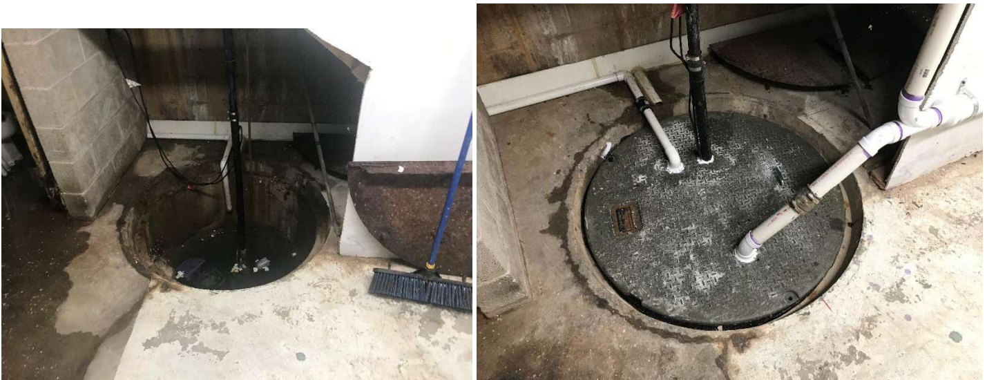
Photo 8. Ejector pit in south basement, Sump S3, before and after sealing.
