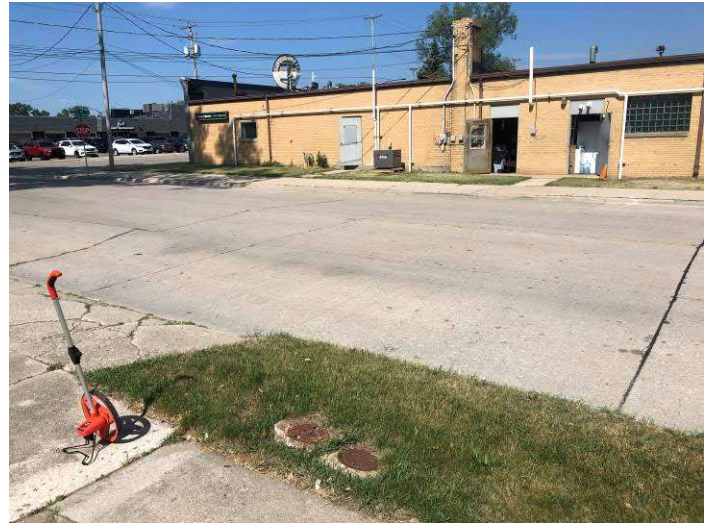
Photo #2 View of outdoor vent piping and fans facing southwest.
