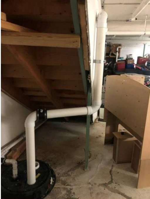
Photo #9 View of Sump 4 facing southeast.
