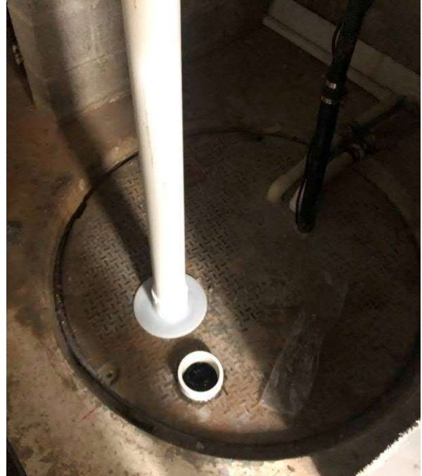
Photo #10 View of Sump 3 facing southeast.
