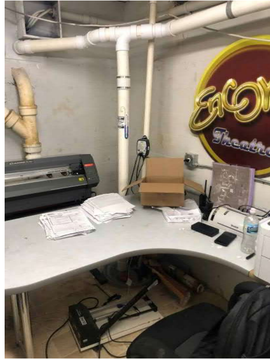
Photo #8 View of Sump 1 and differential pressure gauge facing northwest.
