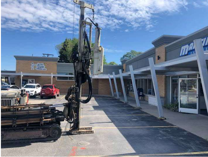
Photo #11 View of installation of monitoring well MW-4R facing northeast
