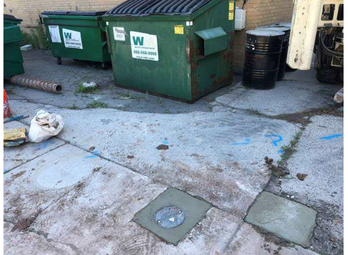
Photo #12 View of monitoring well MW-7R facing west.
