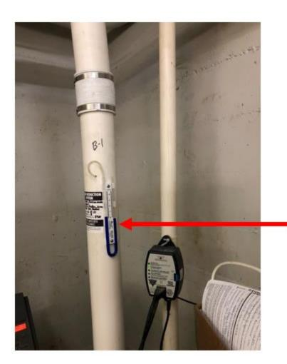
Pipe labeled "B-1" in southern basement has manometer reading of only 0.2" WC
