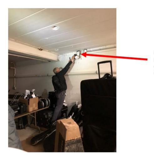
Capped pipe entering basement that may b entry point for vapors elevated detections o
