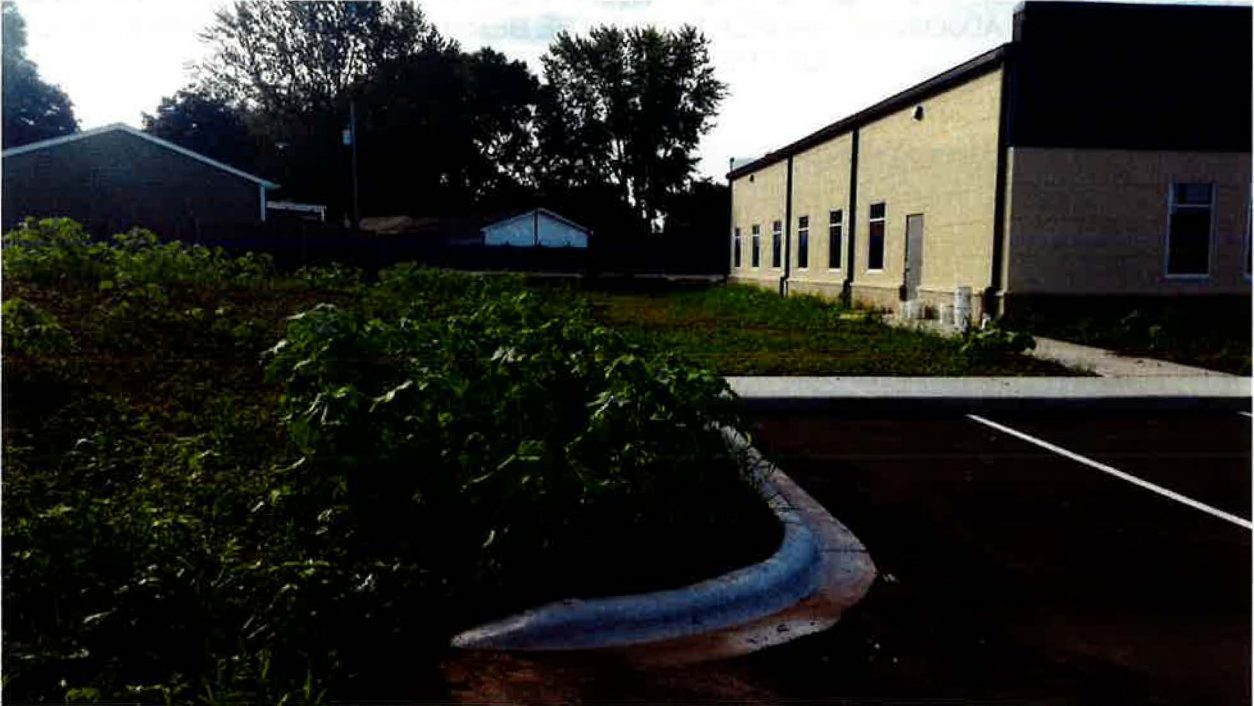
PHOTOGRAPH OF BERM AREA ALONG THE NORTHEASTERN PORTION OF THE PROPERTY VIEWING TOWARD THE SOUTHEAST
