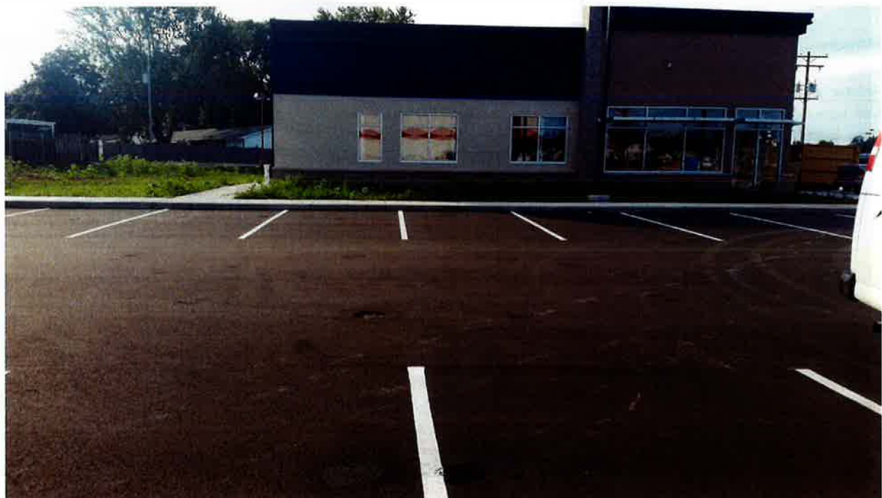
PHOTOGRAPH OF PAVED AREA AROUND MW-4 VIEWING TO THE SOUTHEAST TOWARD THE FAMILIA DENTAL BUILDING
