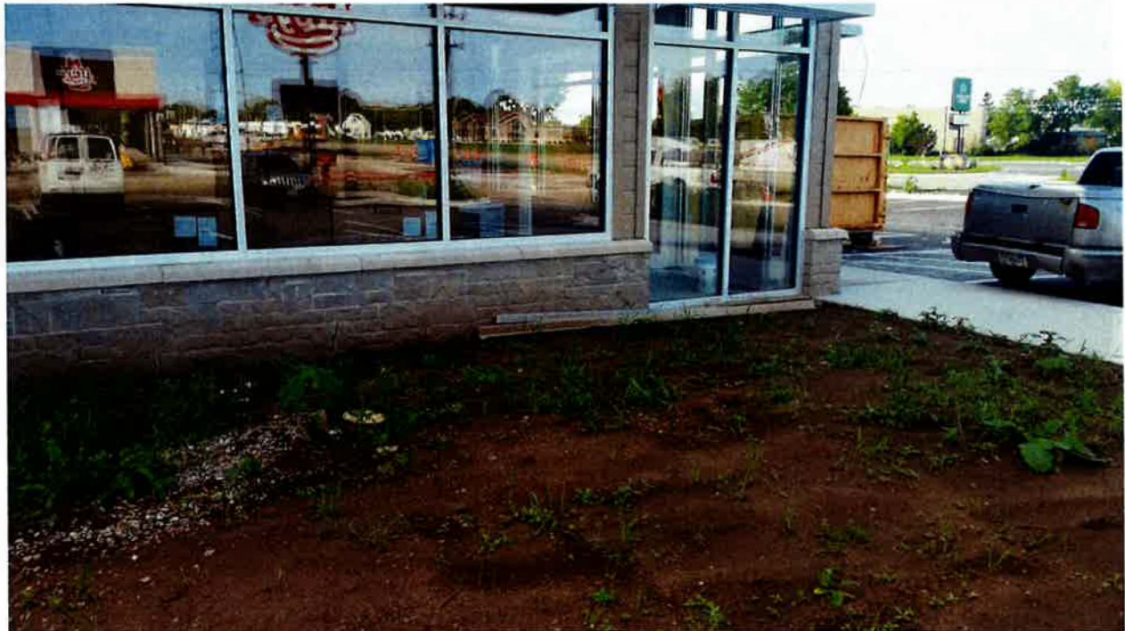
PHOTOGRAPH OF TW-5 NEAR THE SOUTHWESTERN PORTION OF THE FAMILIA DENTAL BUILDING
