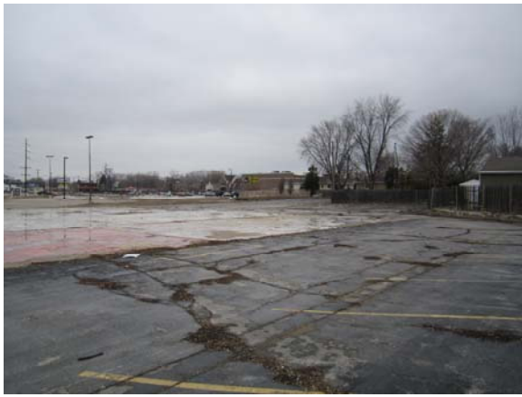
Photo 7: Post building demo, face North from eastern property line (April 2014)
