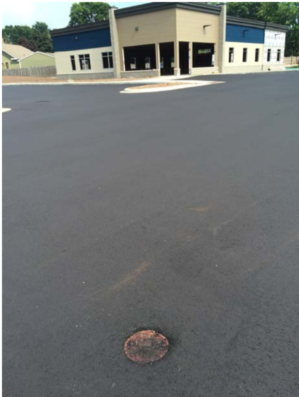
Photo 11: Redevelopment building after asphalt laid, face East from near MW-9 (August 2016)
