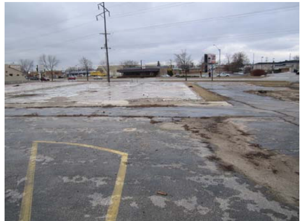
Photo 6: Post building demo, face South near MW-4 (April 2014)
