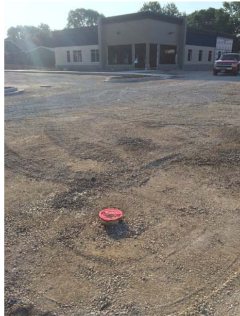
Photo 10: Redevelopment building, face East from near MW-9 (August 2016)
