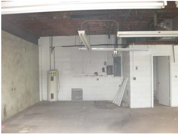
Photo 3: Pre building demo, inside building, face Southeast from Northwest wall (July 2012)
