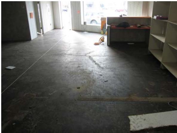
Photo 5: Pre building demo inside drilling, face South near GEC TW-1 (December 2012)
