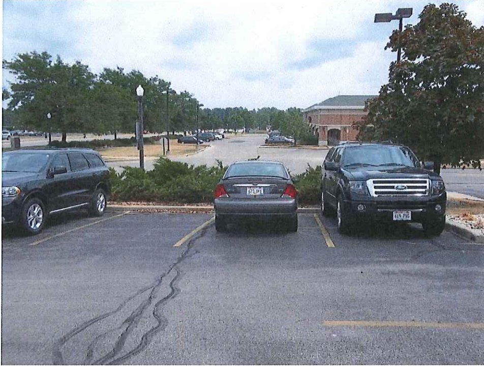
Looking east at the east portion of the asphalt cap
