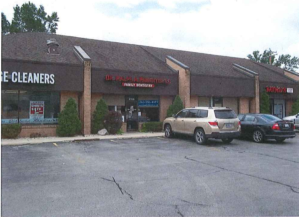
Looking south at the northwest portion of the asphalt cap
