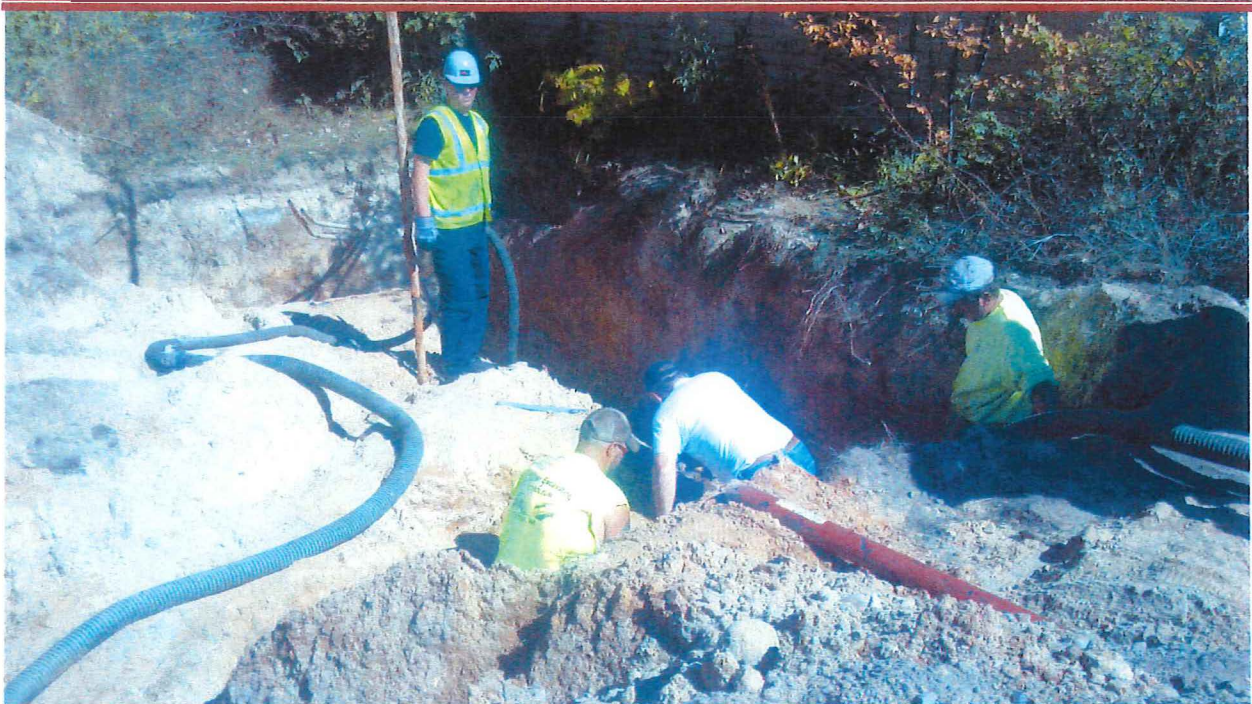
PHOTOGRAPH OF PUMPING OF THE TANK EXCAVATION AND PUMPING OF TANKS
