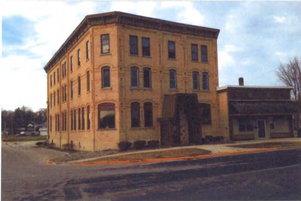
Photo 1: Central House building
