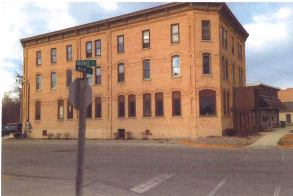
Photo 2: Central House building
