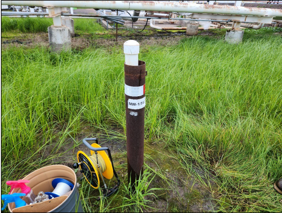
Photo 1: MW-1/T40 before riser was replaced. Photo taken on October 16, 2023.
