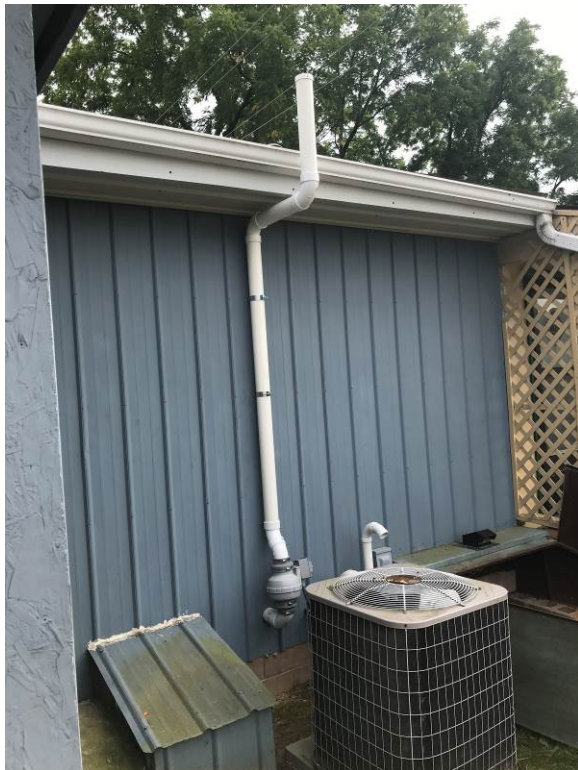
Photo 6: Fan and exhaust line Date: 8/14/2018
