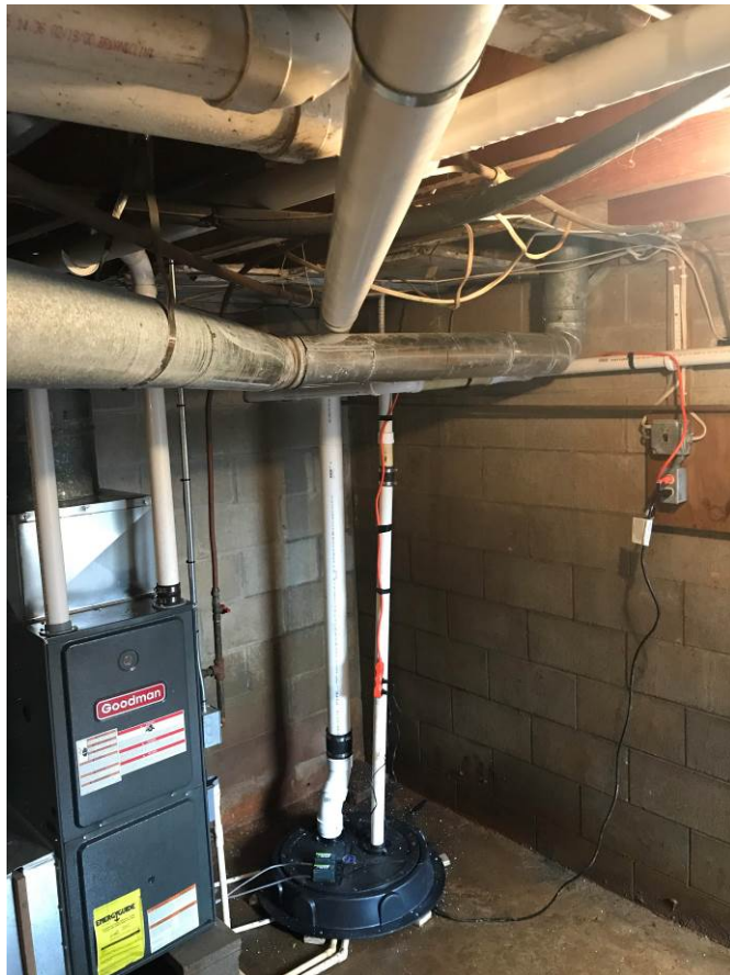
Photo 4: Pick-up point and piping Date: 8/14/2018
