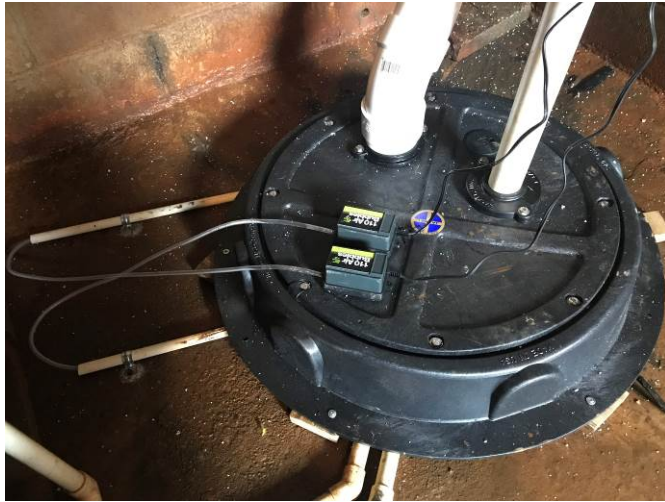
Photo 3: Sump lid with aeration pumps Date: 8/14/2018
