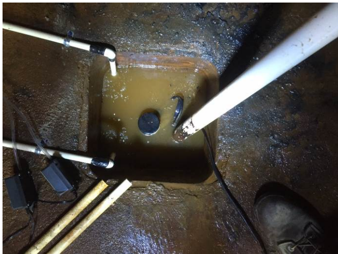
Photo 2: Sump pit with aeration system installed Date: 8/14/2018
