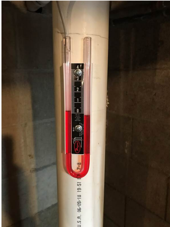
Photo 5: Pick-up point manometer Date: 8/14/2018
