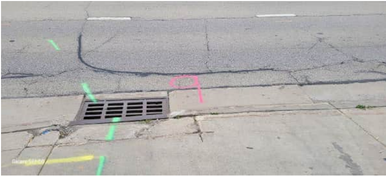
Proposed location of boring B-9 (not completed due to utilities)
