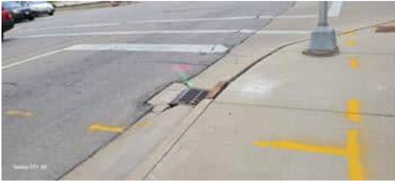
Location of boring B-16a on Cecil Street at the northwest corner of South Commercial Street and Cecil Street adjacent to storm catch basin.
