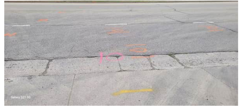
Proposed location of boring B-10 (not completed due to utilities)
