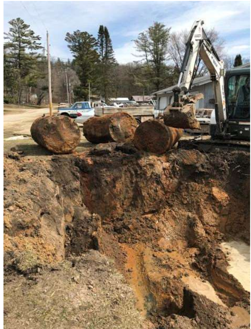
PHOTO 4 - Tanks by Excavation - looking east
