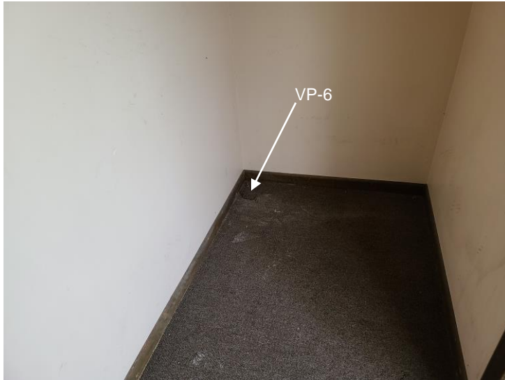
VP-6 is approximately 4 ½ from the exterior wall to the right.
