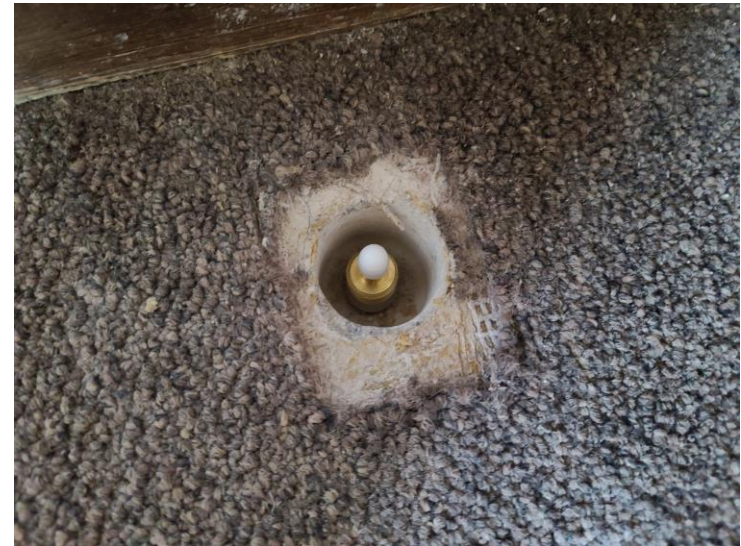
Installed vapor pin.
