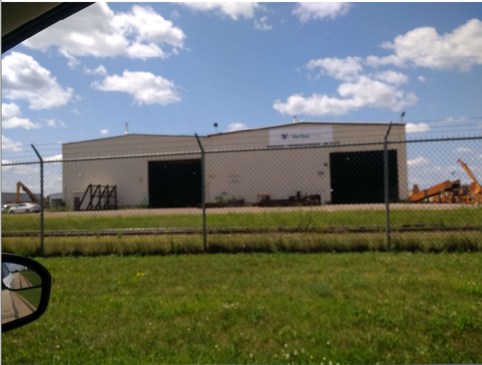
Title: Structural Impediment (Bridge Plant Building) Looking West
