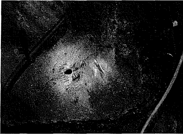
VP-1 location, adjacent to multiple cracks in concrete
