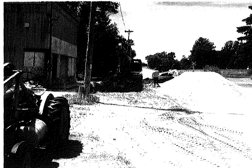
Backfilling of Excavation Area Facing West
