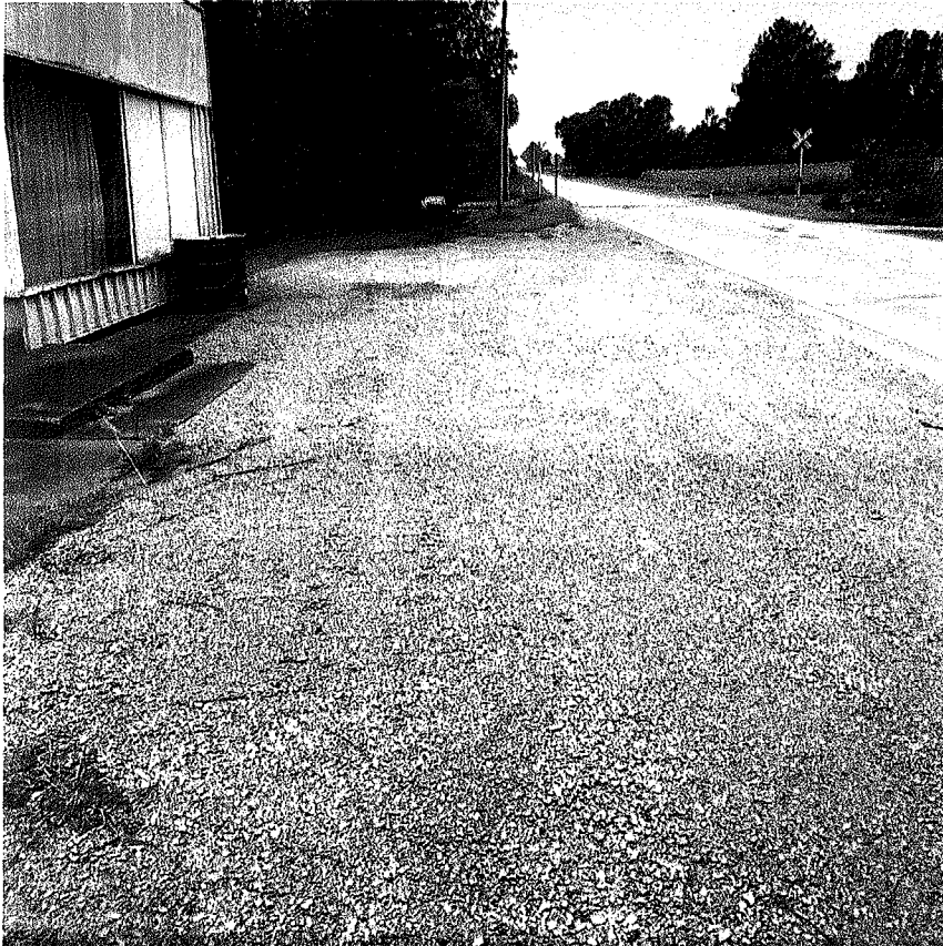
Post Excavation Facing West
