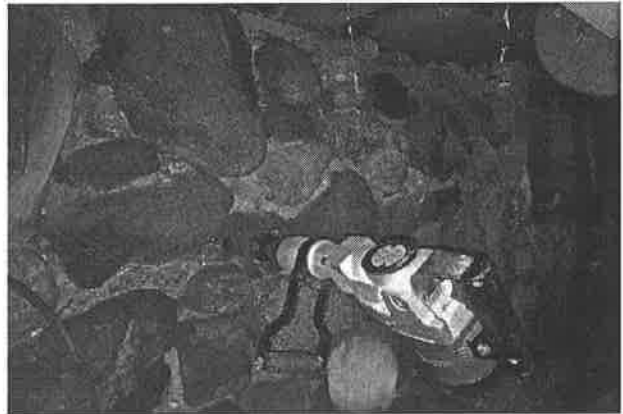
Drilling hole through north wall
