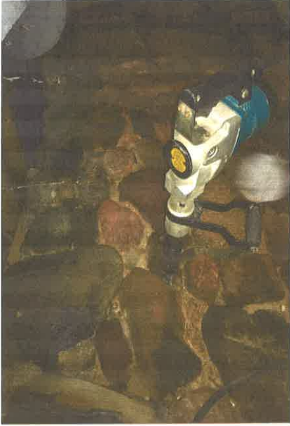
Drilling hole through north wall
