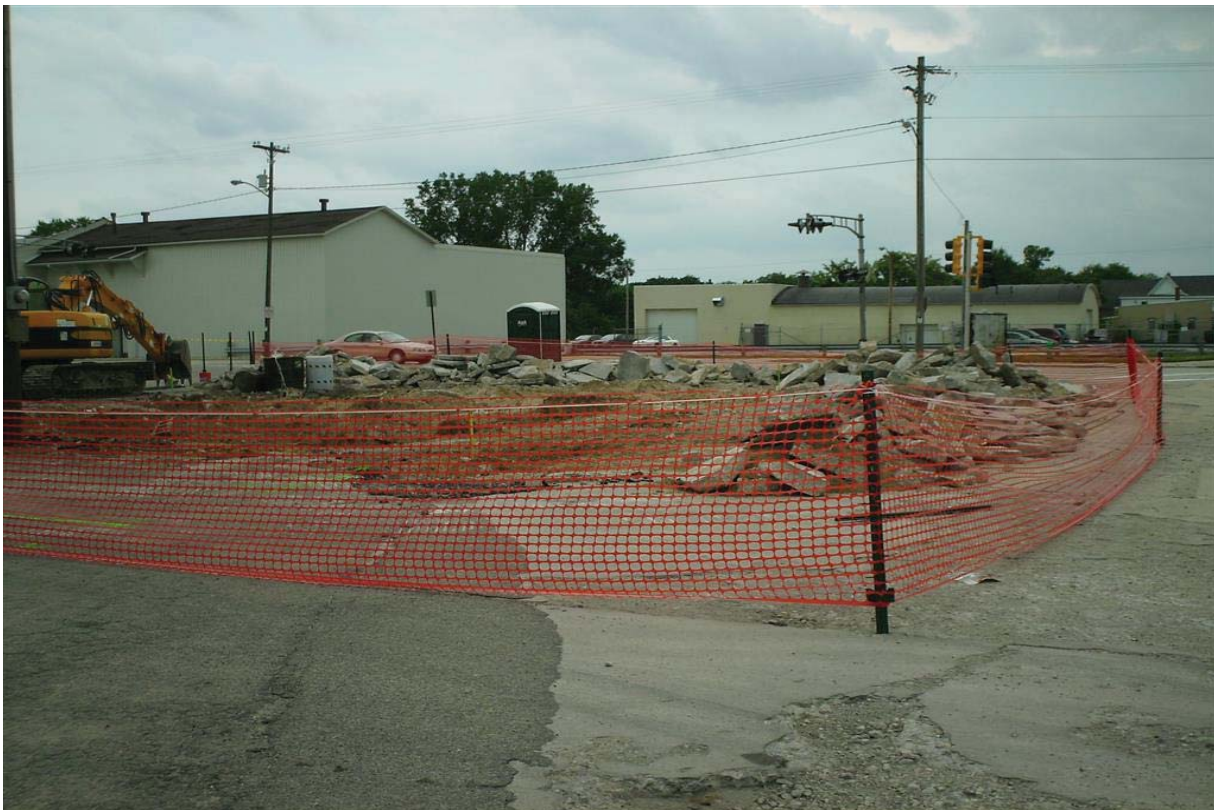
Figure 2. Original building demolished/west view.
