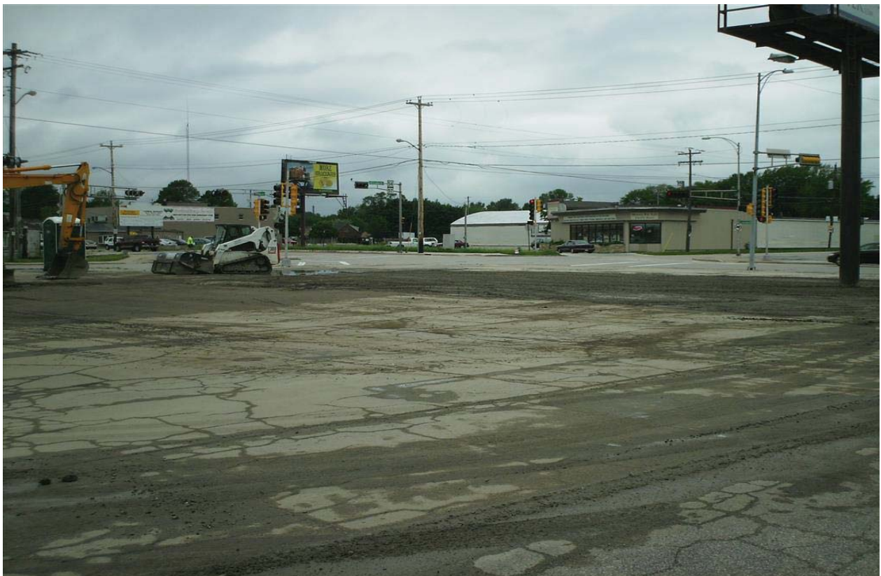
Figure 4. Excavation backfilled/northwest view.
