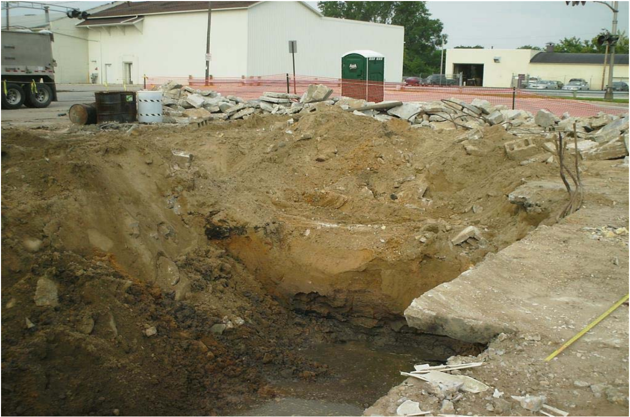
Figure 3. Site excavation/southwest view.
