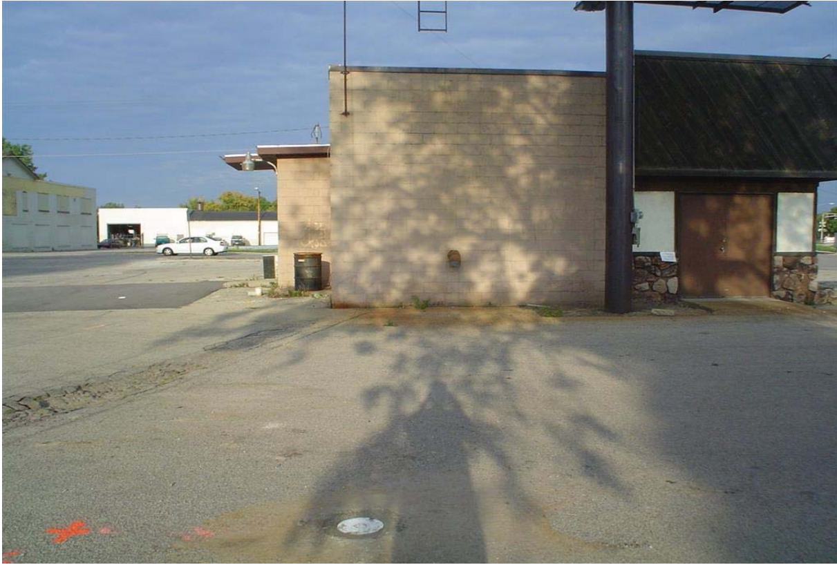
Figure 1. Original site building /west view.
