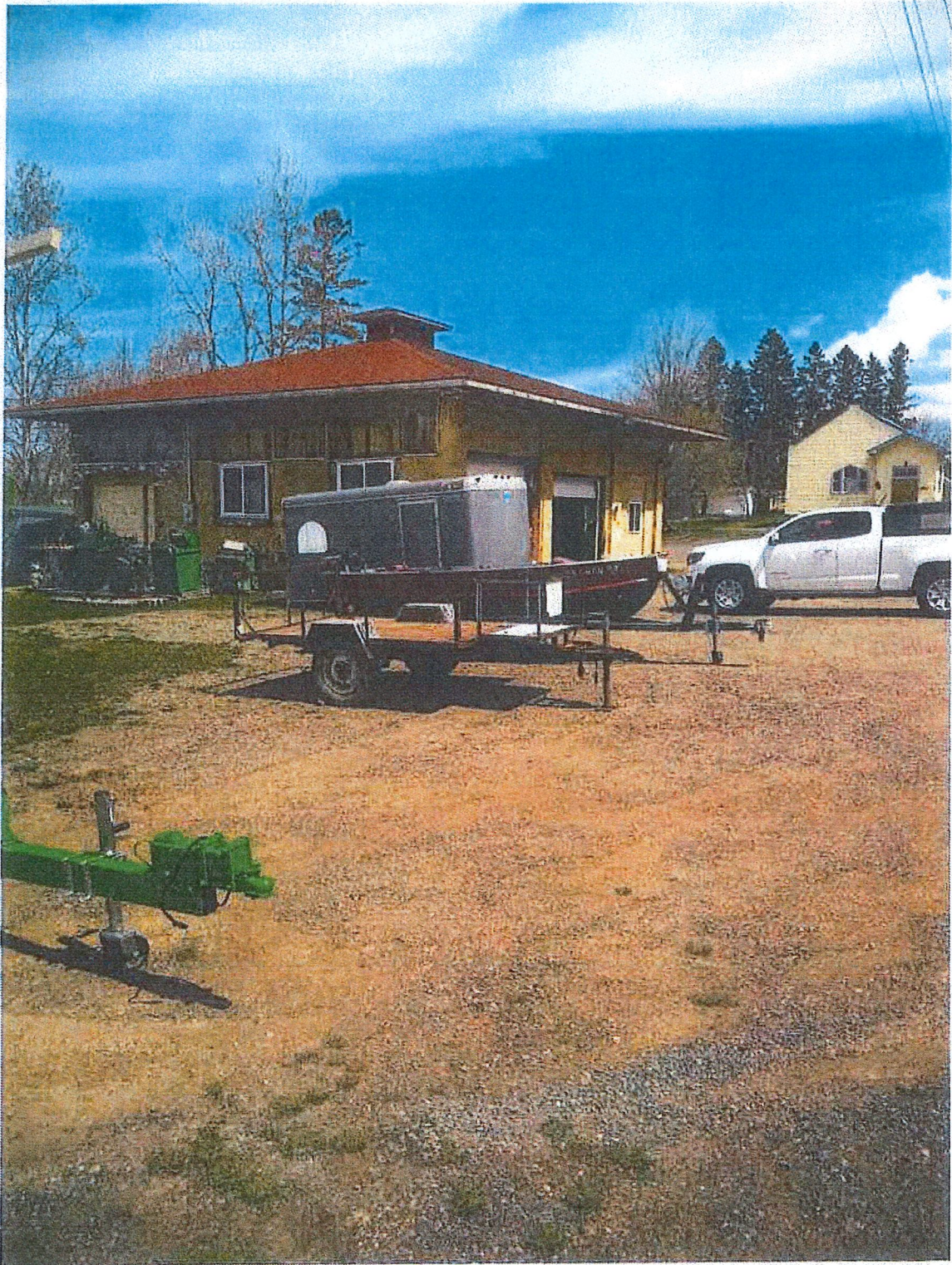
Photo #2: On site building looking East.
