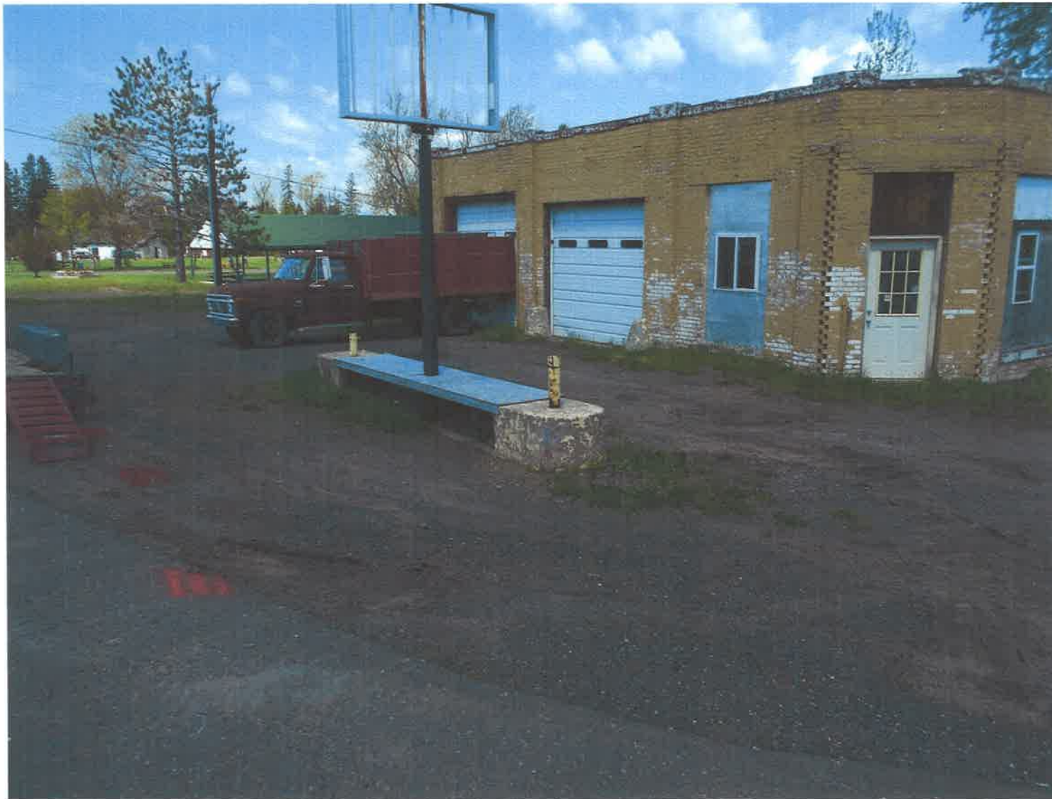
Photo #1: On site building looking west.
