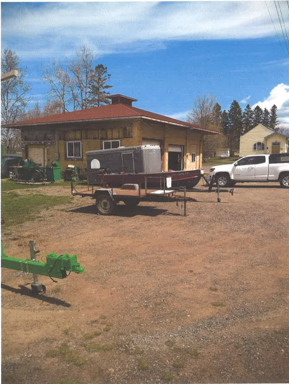
Photo #2: On site building looking East.
