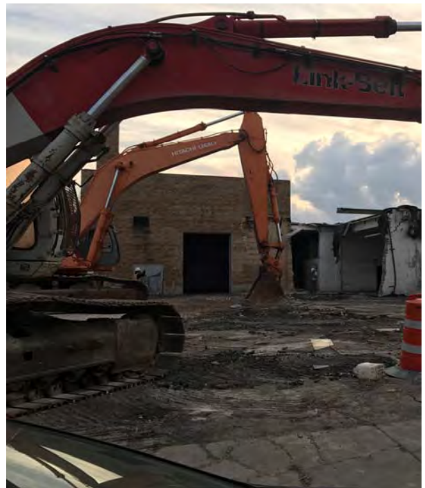
Photo 4: Bay Towel building demolition.
