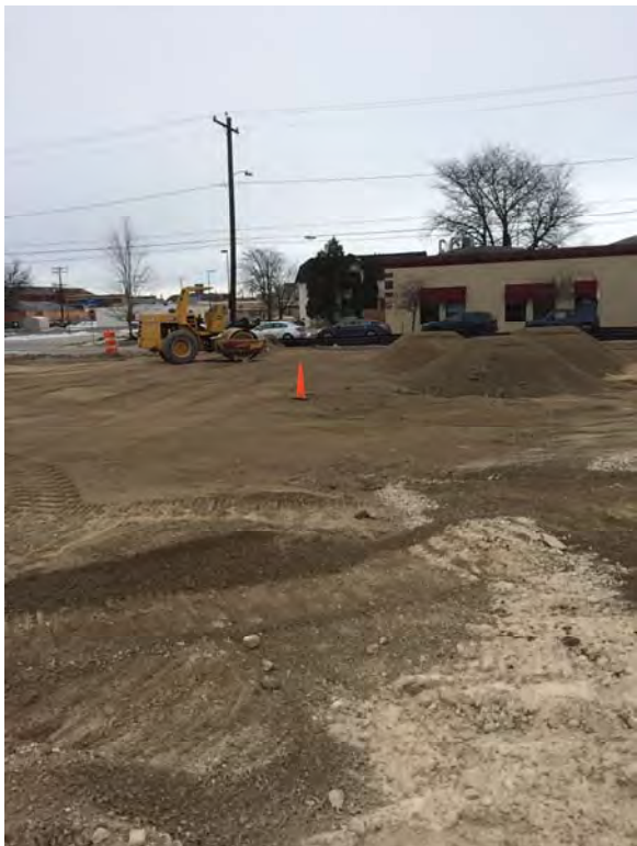
Photo 19: Excavation area after completion of backfilling, looking northeast.
