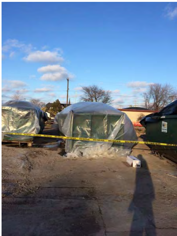
Photo 11: Treated soil stored in roll off containers.
