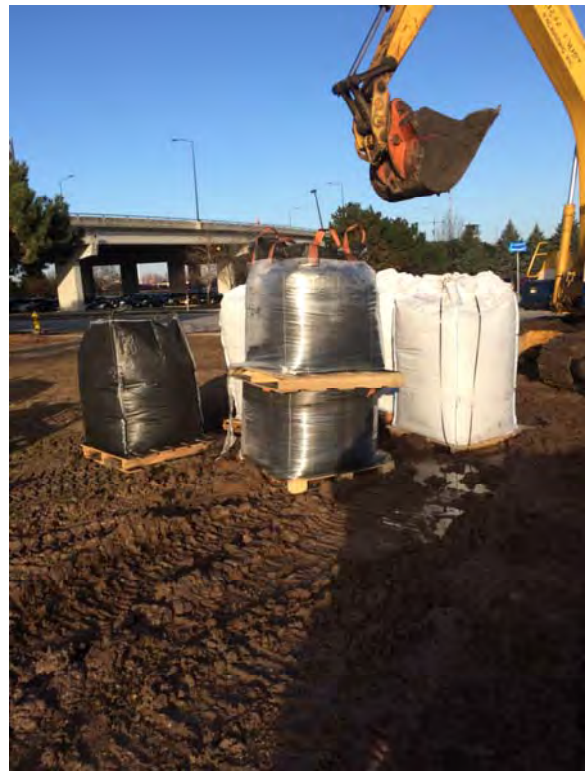
Photo 22: Retreatment of soil in roll off boxes.
