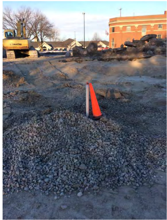
Photo 18: New well SMW-1 installed during backfilling.
