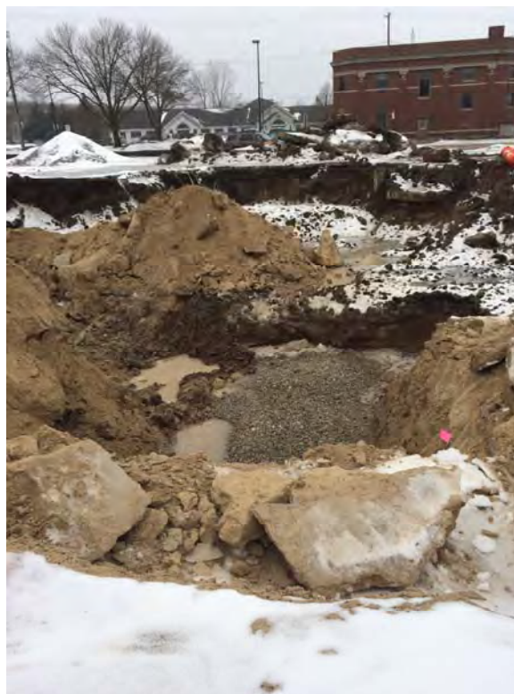
Photo 16: Excavation at 14 feet below ground surface looking west.
