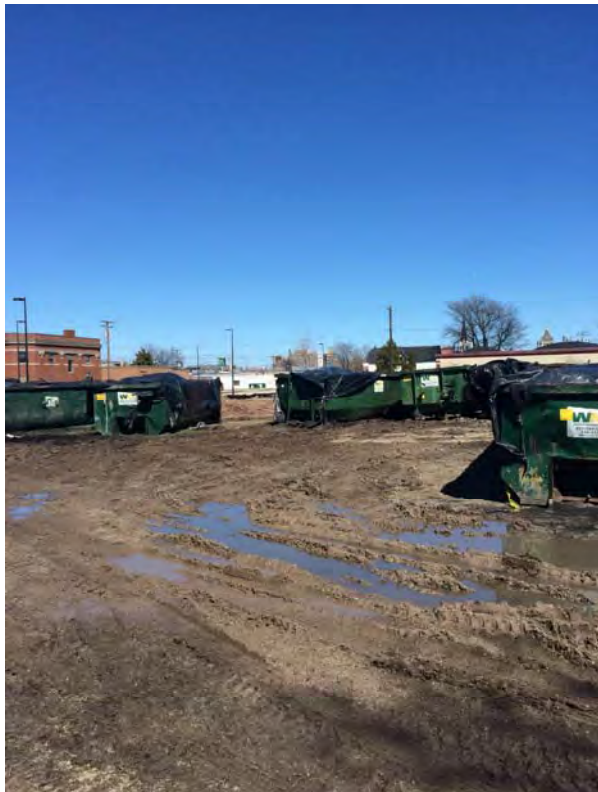
Photo 23: Covered retreated soil in roll off boxes.
