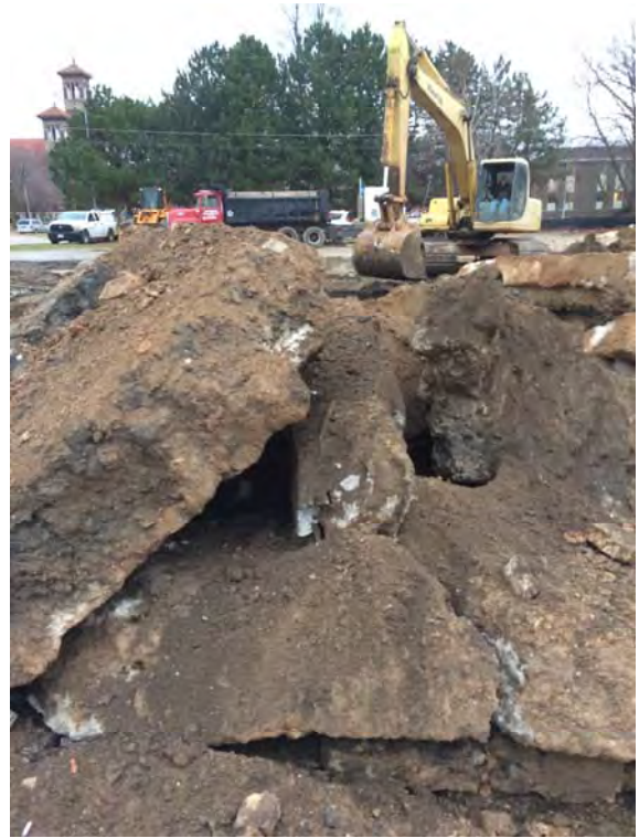
Photo 8: Concrete removed during excavation.
