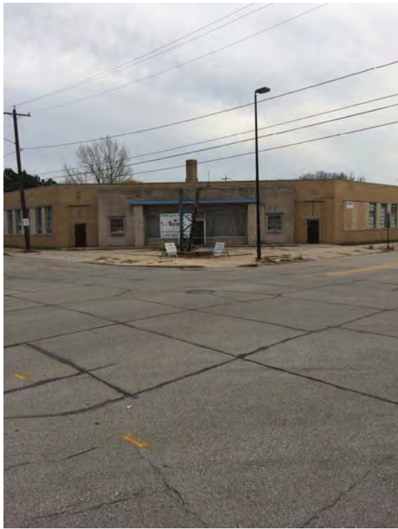
Photo 1: Bay Towel building pre-demolition. Looking south from Chicago Street-Adam Street intersection.
