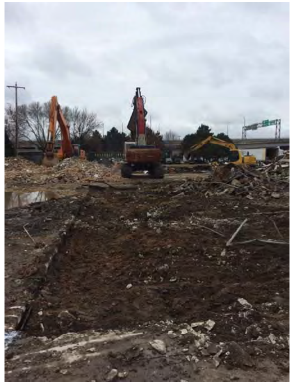
Photo 6: Concrete removal before excavation looking southwest.
