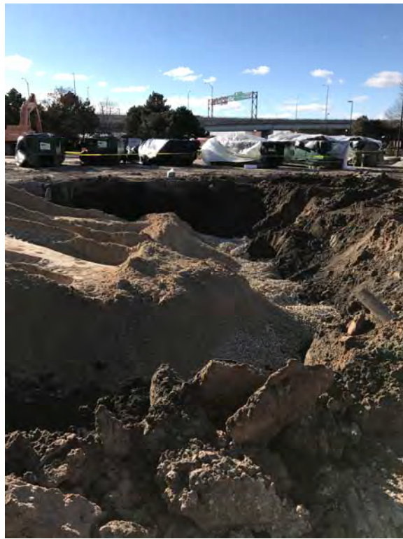
Photo 14: Excavation area looking west.
