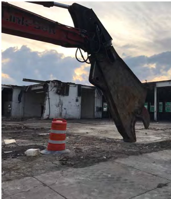
Photo 3: Bay Towel building demolition.
