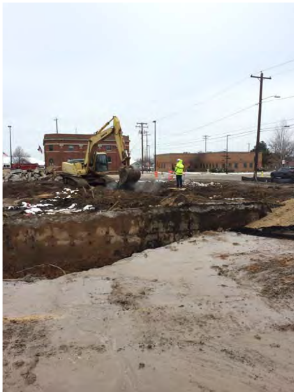
Photo 9: Soil treatment and mixing with Fentons and BAM.
