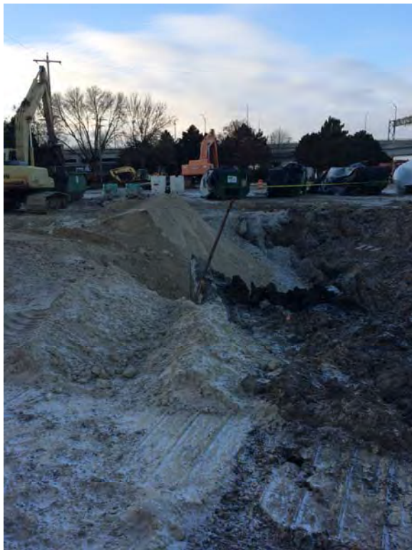
Photo 13: Excavation with start of backfilling.
