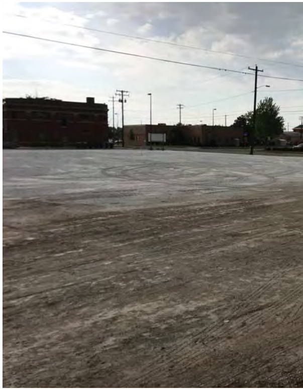
Photo 26: Final grading of site, looking north.
