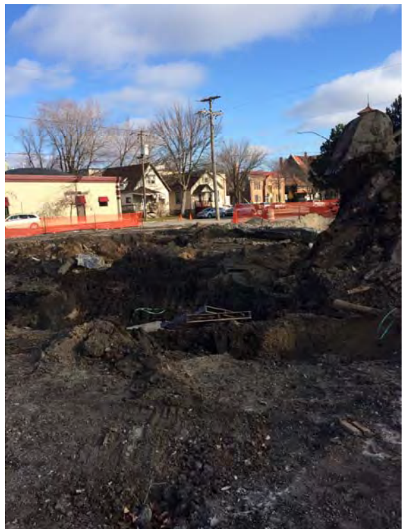
Photo 12: Excavation after soil treatment, looking east.
