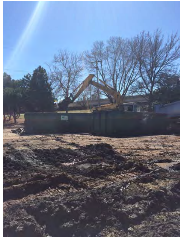
Photo 24: Disposal of retreated soil to landfill.
