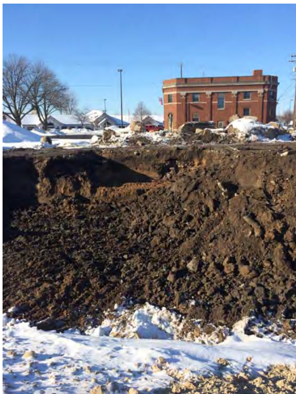
Photo 15: Excavation area looking northwest.
