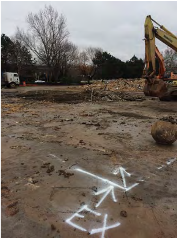
Photo 5: Concrete removal before excavation looking south.
