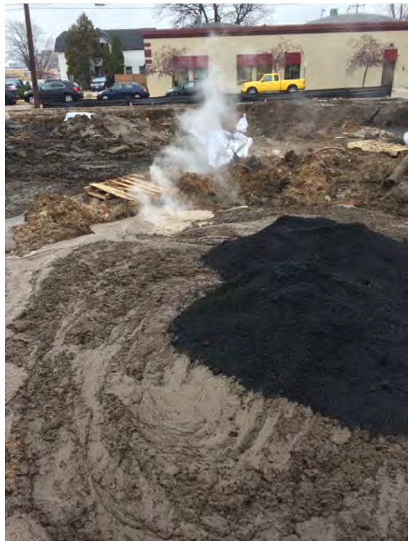
Photo 10: Soil treatment and mixing with Fentons and BAM.
