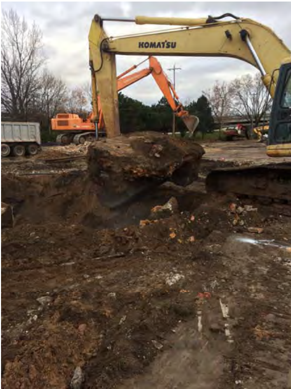
Photo 7: Old house foundation removal during excavation.
