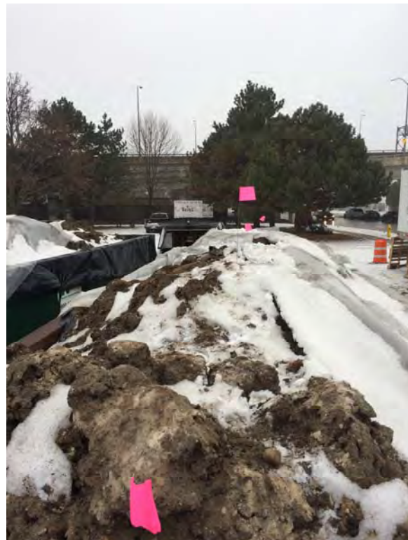
Photo 20: Sampling of treated soil in roll off boxes post-excitation.
