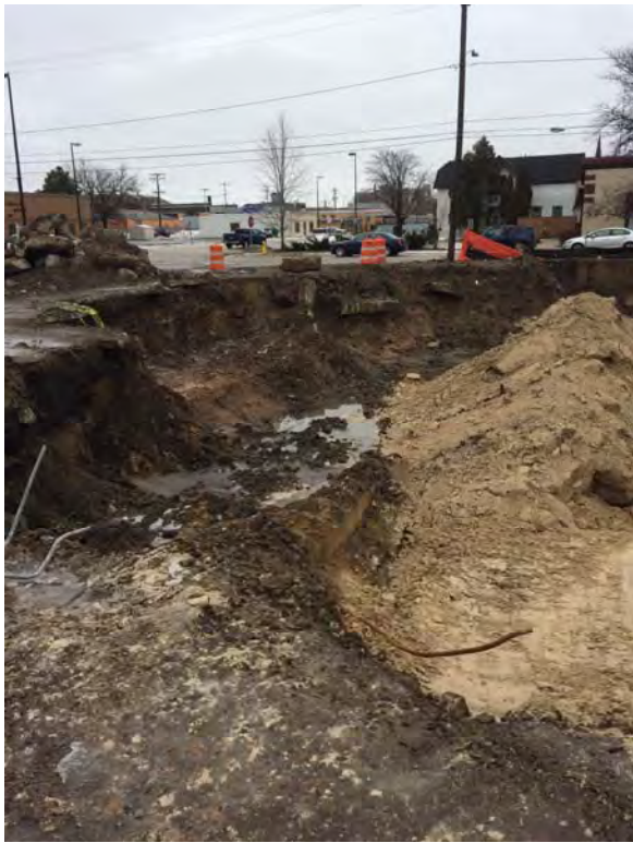
Photo 17: Excavation area looking north.
