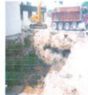
CONTAMINATED SOIL EXCAVATIONS
