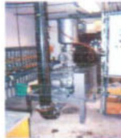
REMEDICATION SYSTEM CONSTRUCTION
