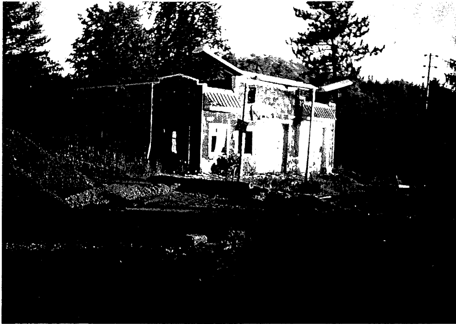
Photograph #1: View of the former Thomas service station (facing southwest).
