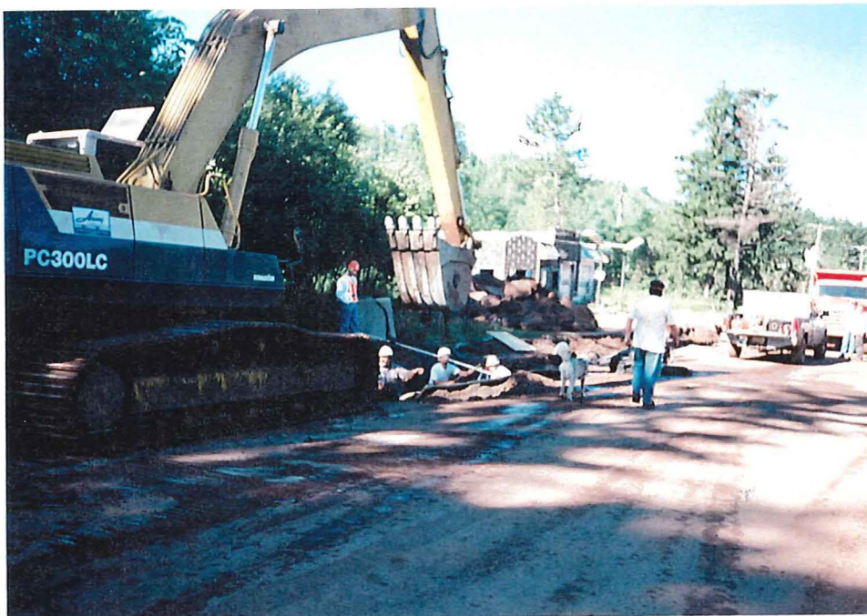
Photograph #4: View of the excavation and transportation equipment.
