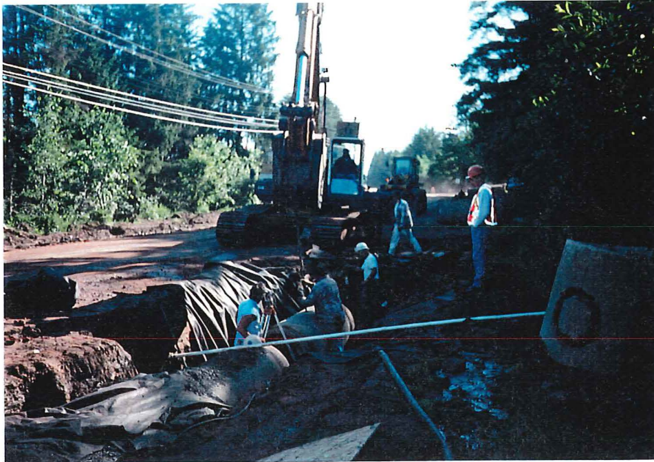
Photograph #5: View of storm sewer installation activities (facing northeast).
