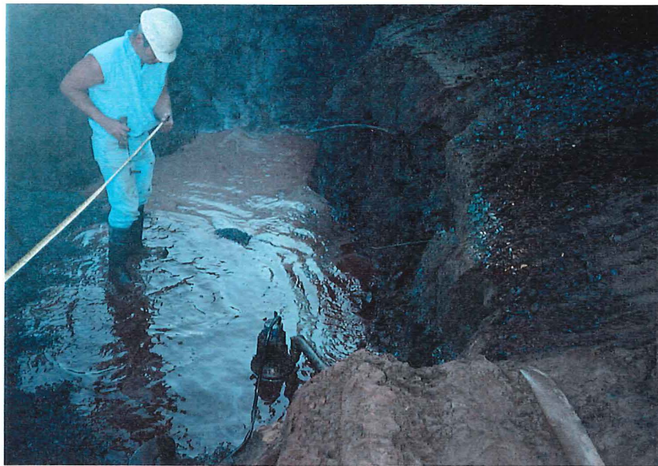
Photograph #6: View of dewatering activities in installing the storm sewer.
