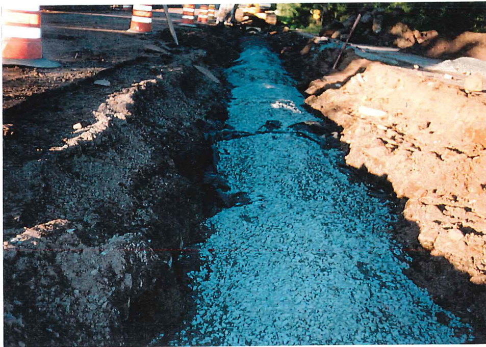
Photograph #7: Closer view of the installed storm sewer (facing east).
