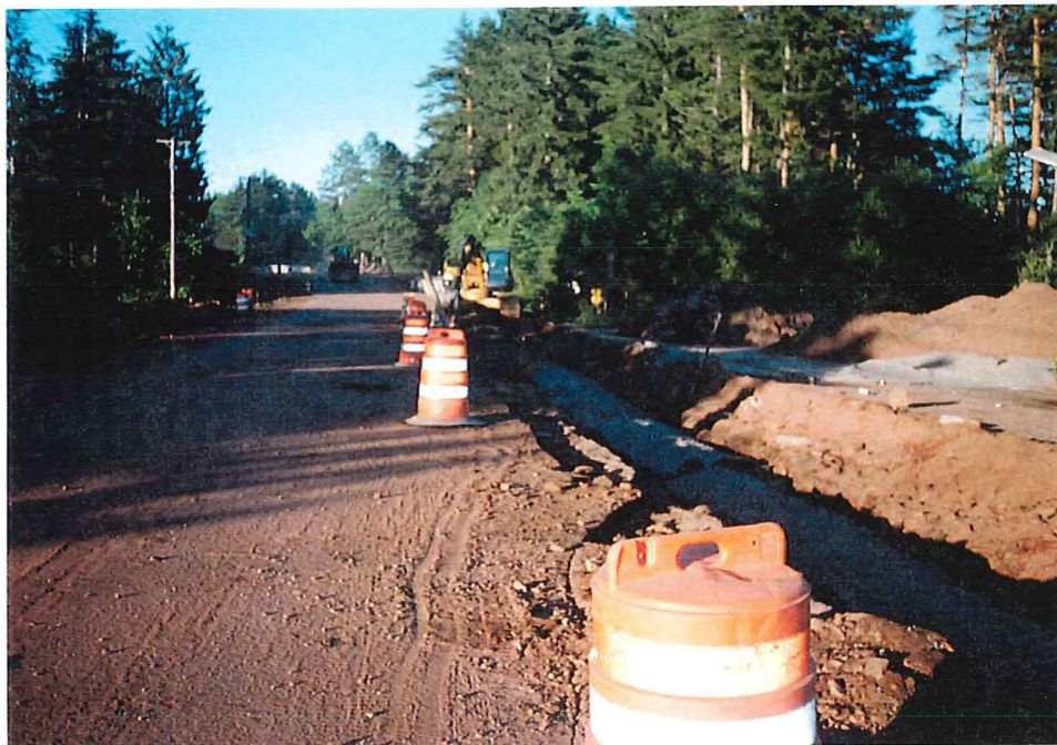
Photograph #8: View of the installed storm sewer (facing southeast).
