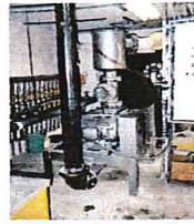
REMEDIAION SYSTEM CONSTRUCTION
