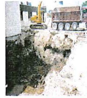
CONTAMINATED SOIL EXCAVATIONS
