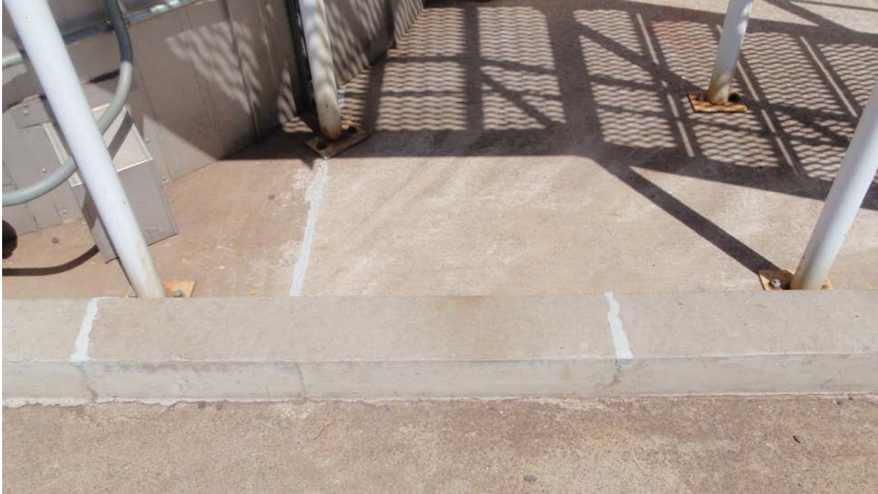
Photo 2 – show concrete cap in good shape, with attached structures
