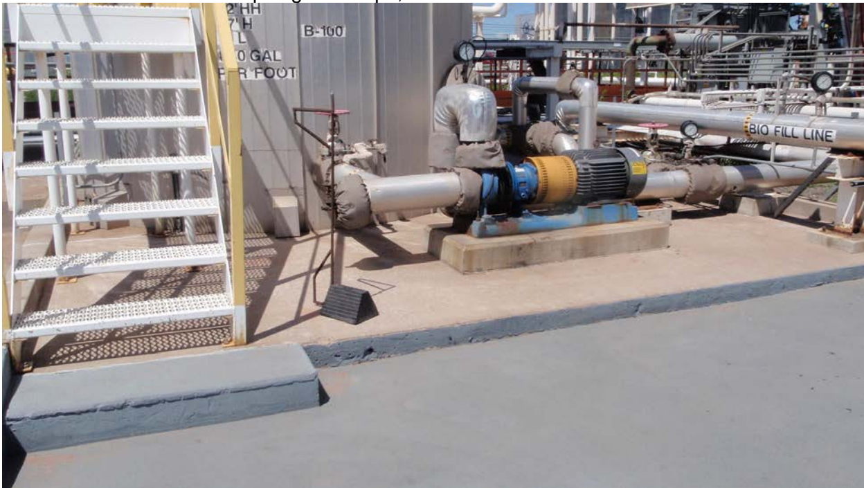
Photo 2 – show concrete cap in good shape, with attached structures
