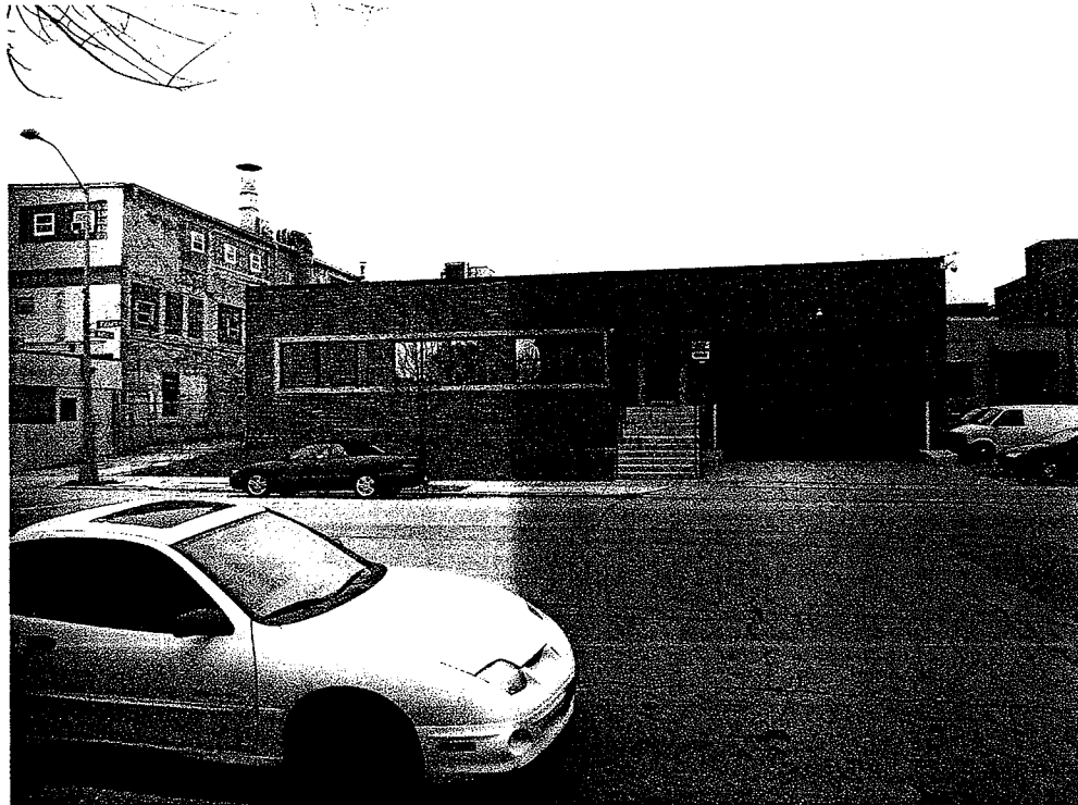
Photo 5: Looking west from Packard Avenue at south end of building.
