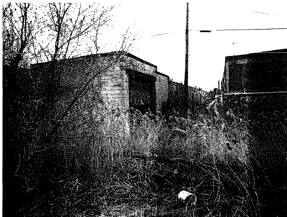
Photo 8: Looking northeast at southwest corner of building.
