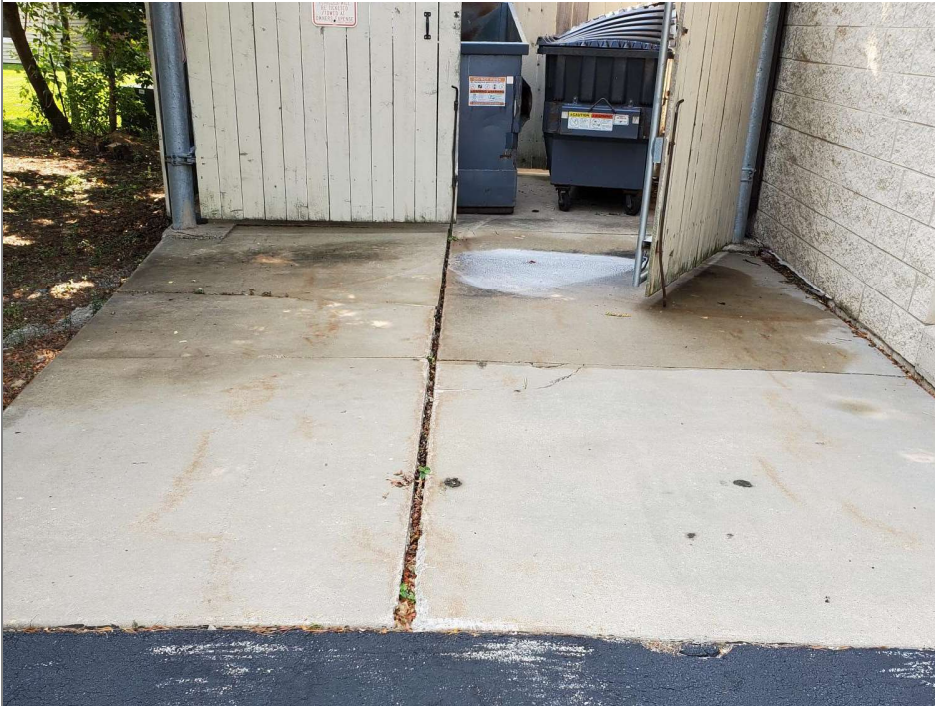
Title: Dumpster area surface, east side of lot
