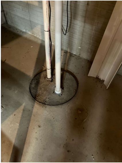
Description: Typical sealed sump
