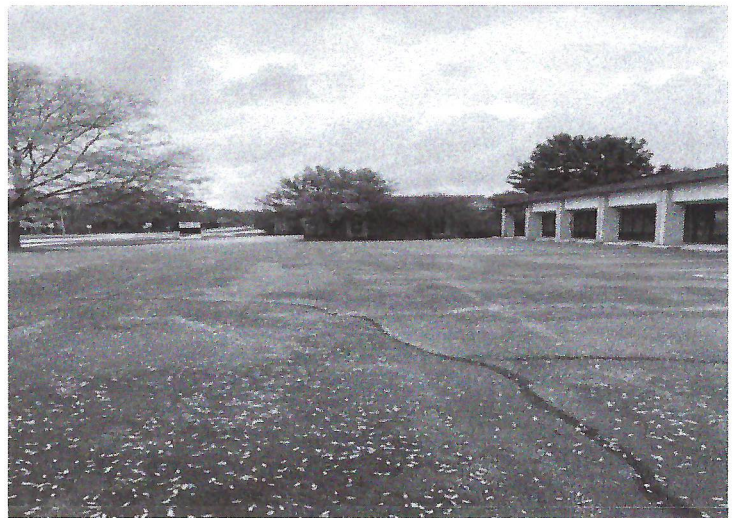
Photo 4. Looking east at existing asphalt pavement. Pavement appears to be in good condition with sign of deterioration or exposed soil.
