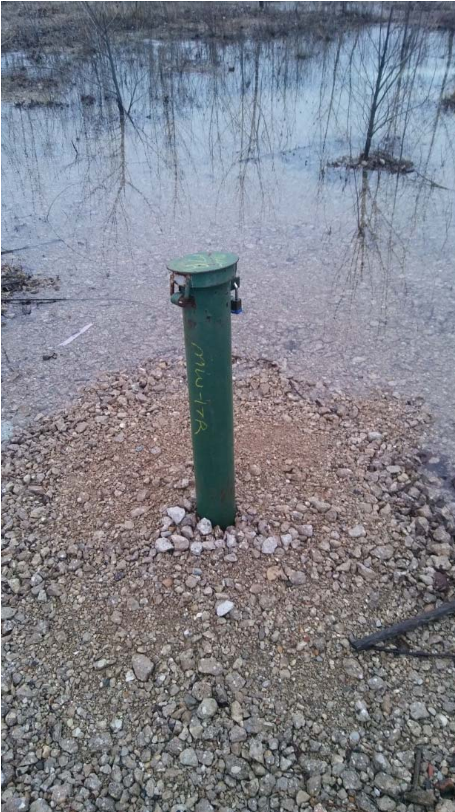
Trent Tube Plant 1 Group A Monitoring Well MW-17R – Photograph taken 1/17/17
