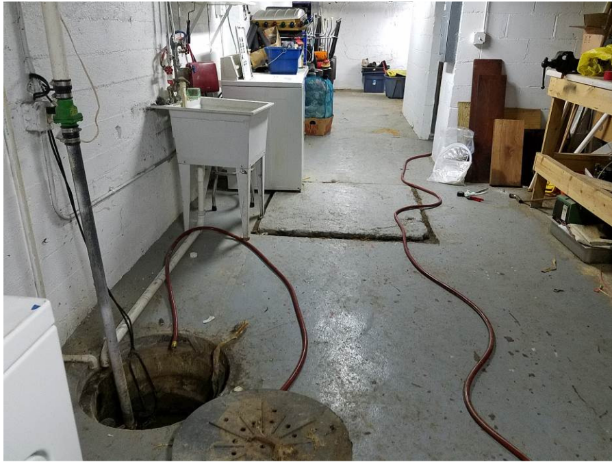
Photo 1: Looking east at sump
