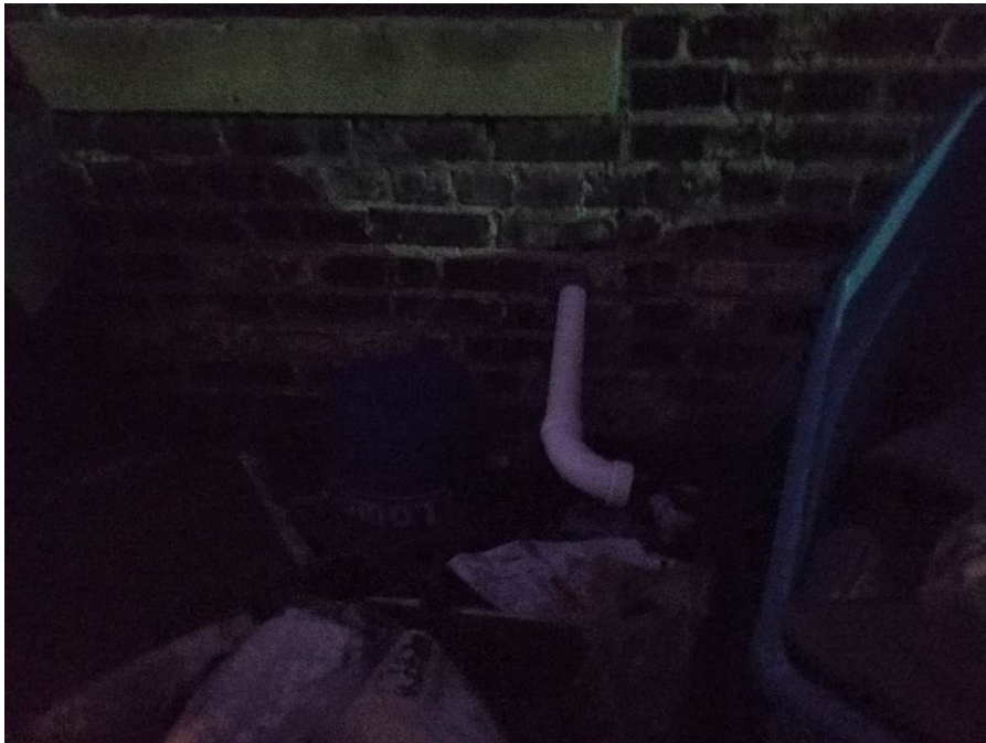
Photo 6: Sump pump discharge point outside east end of building
